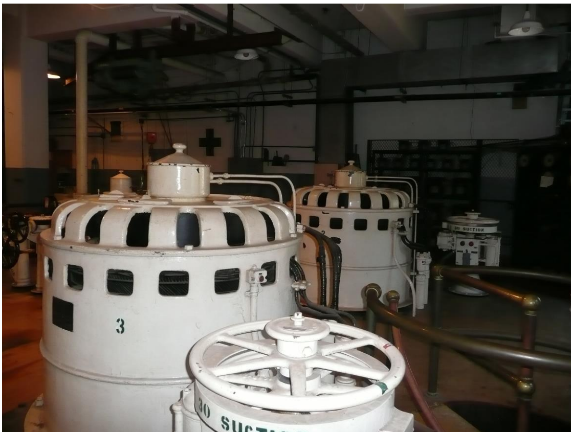
Figure 22–8. Original dewatering pumps and valves, Chittenden Locks, Seattle, Washington
