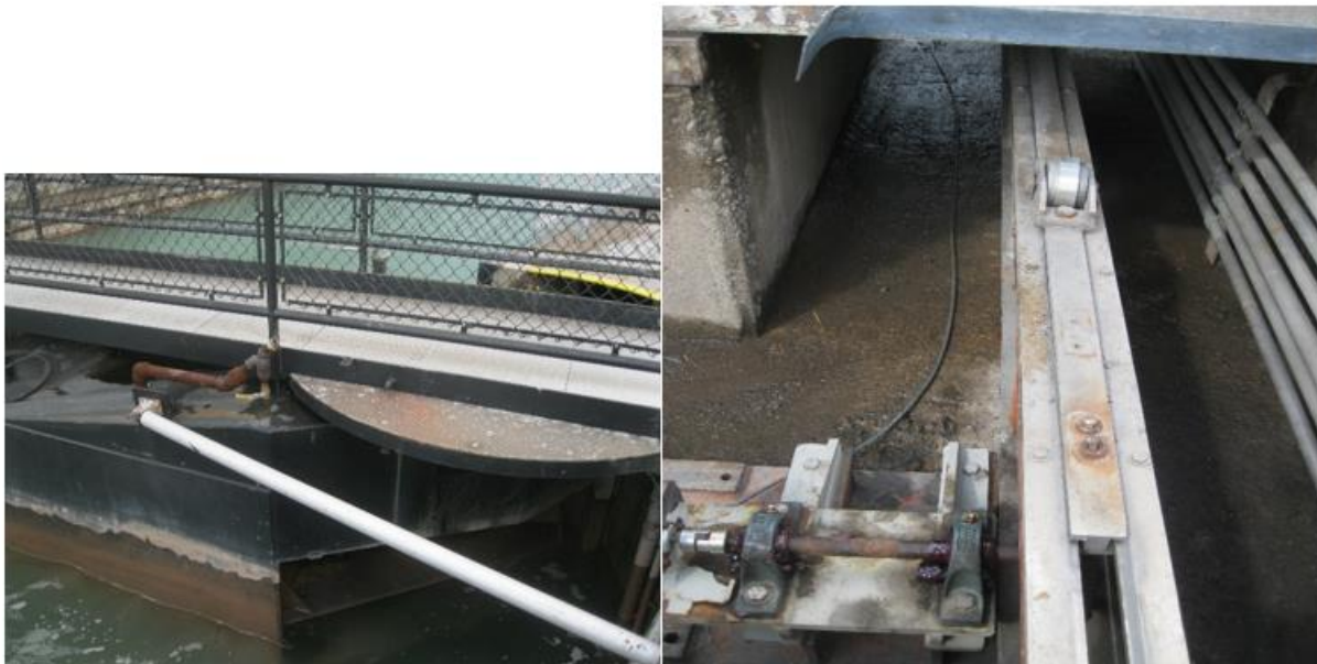
Figure 5–6. Soo Locks miter gate drive train for external position indication
