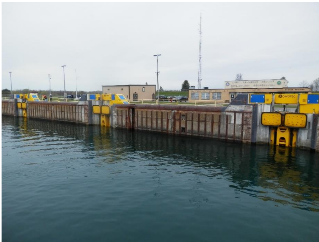
Figure 25–2. Eisenhower Lock Cavotech system
