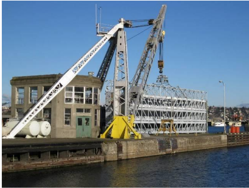
Figure 26–12. Emergency bulkhead crane system, Chittenden Lock, Lake Washington Ship Canal
