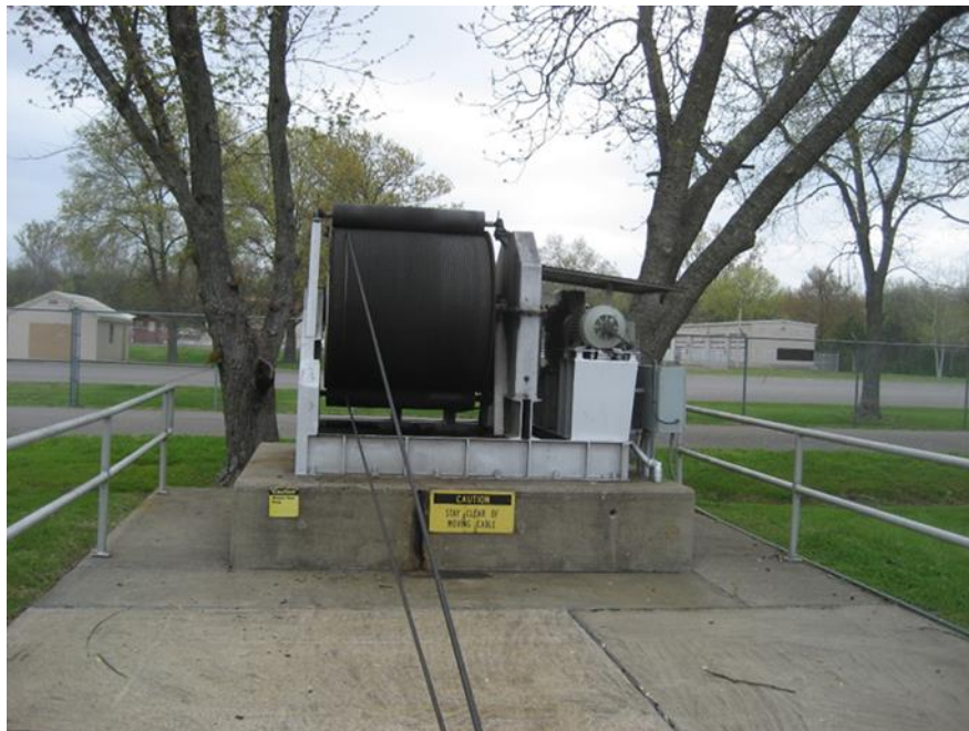
Figure 12–5. Cheatham Lock – original single winch unit with bull gear and pinion
