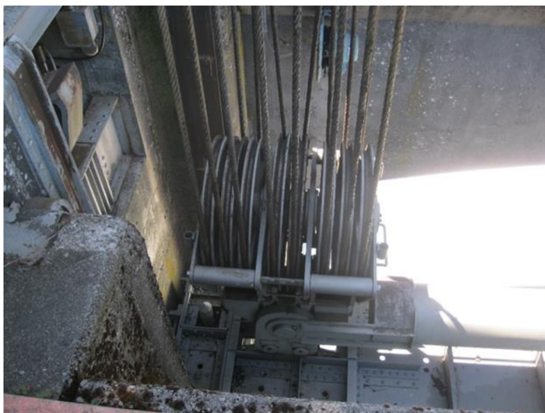
Figure 9–11. Bonneville Dam wire rope and sheaves for vertical gate
