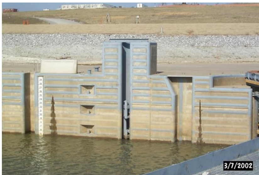
Figure 12-36. Olmsted Lock – floating mooring bitt concrete extension
