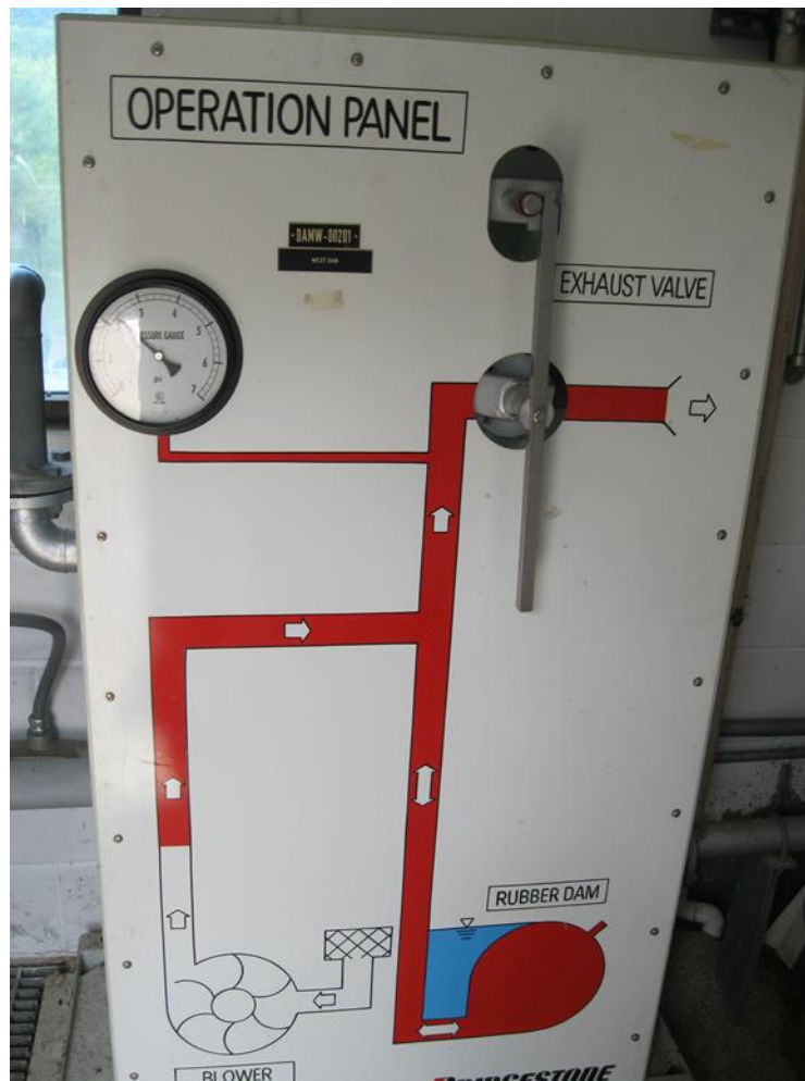
Figure 13–12. Operation Panel – Palmer Dam, Illinois
