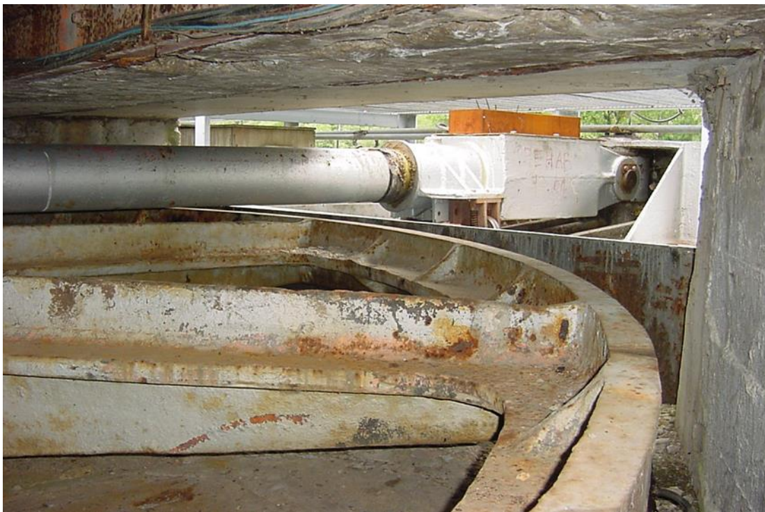
Figure 6–2. Dresden Lock, Illinois River, Panama Canal linkage
