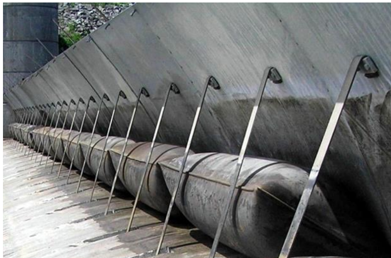
Figure 13–8. Typical steel rubber gate, Saylorville Lake Dam, Iowa
