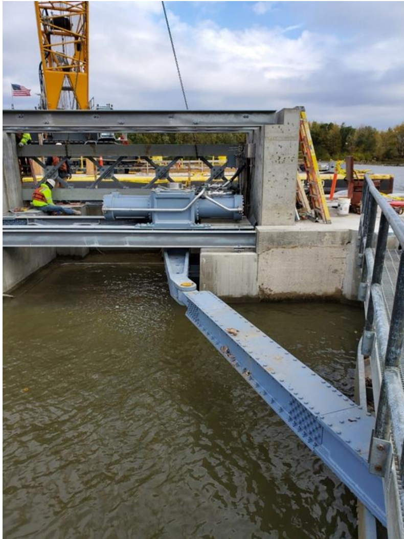
Figure 4–7. Rotary-actuated miter gate machinery La Grange Lock
