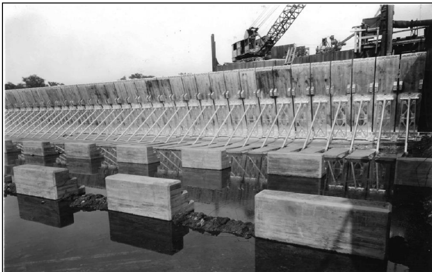
Figure 24–1. Manually operated wicket gates in the raised position (viewed from the downstream side)
