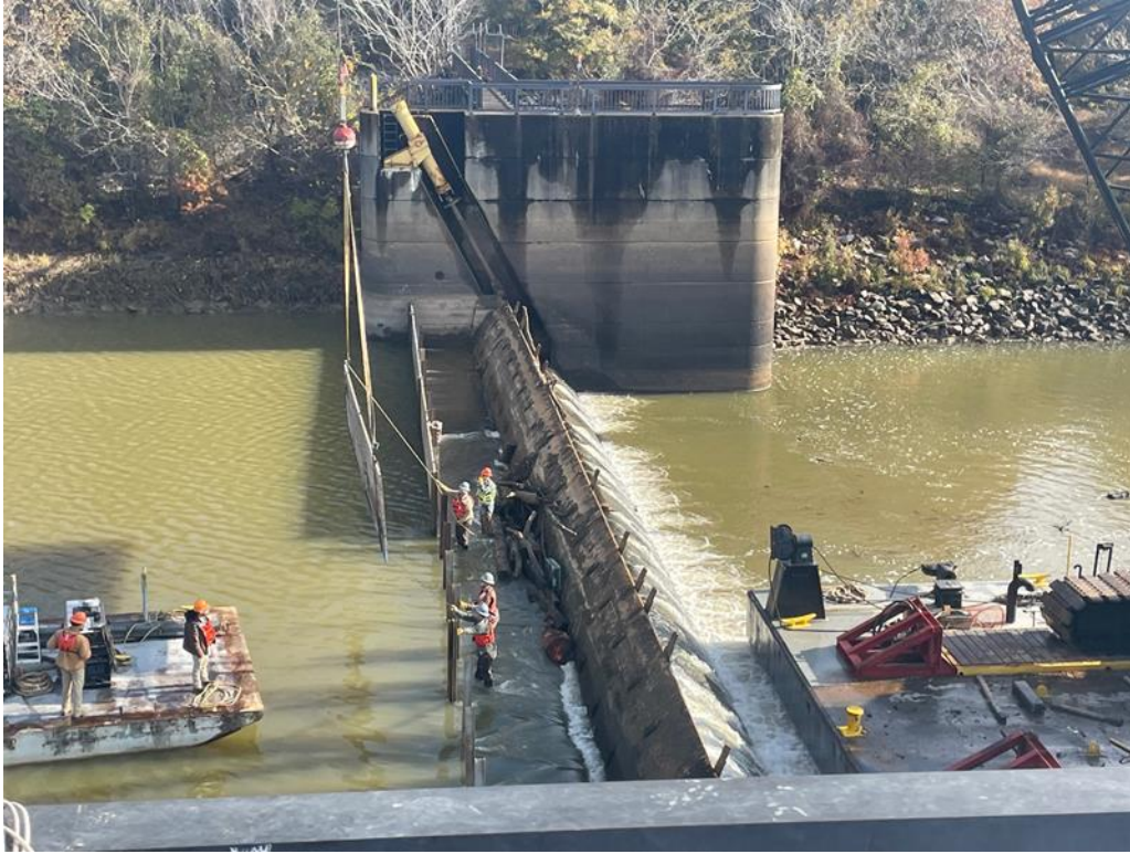
Figure 11–25. H.K. Thatcher torque tube-style hinged crest gate
