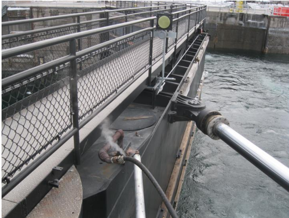
Figure 6-9. Direct-connected linkage for miter gate, Soo Locks
