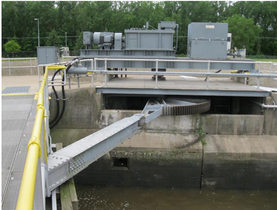
Figure 1-1. Electromechanical drive system at Lock 2 on Mississippi River
