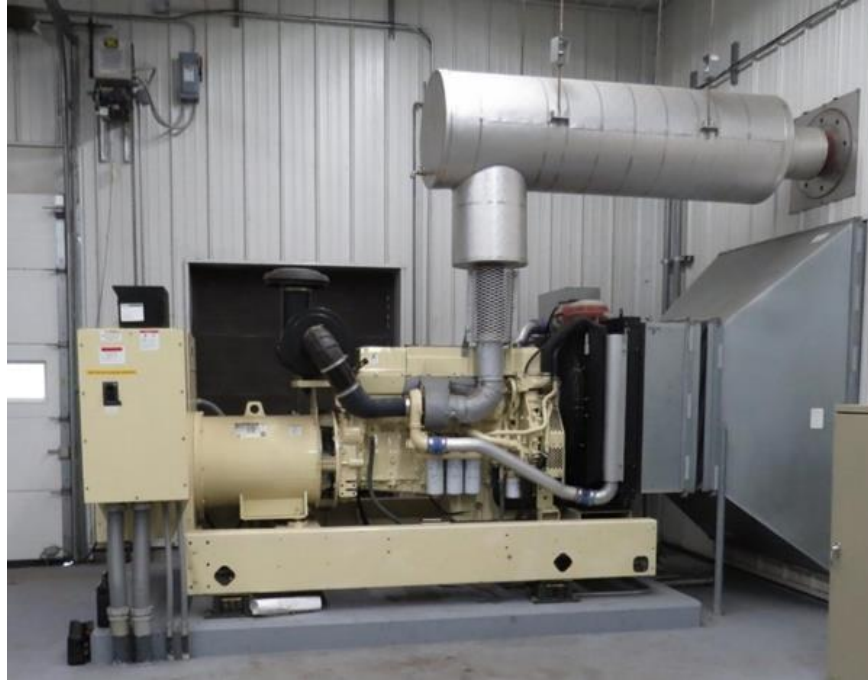
Figure 15–7. Standby diesel generator supplied by external fuel tank at a lock
