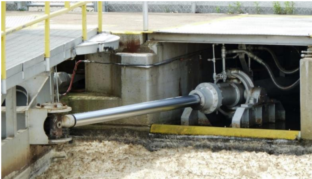
Figure 5–2. Lower St. Anthony Falls Lock hydraulic cylinder for miter gate
