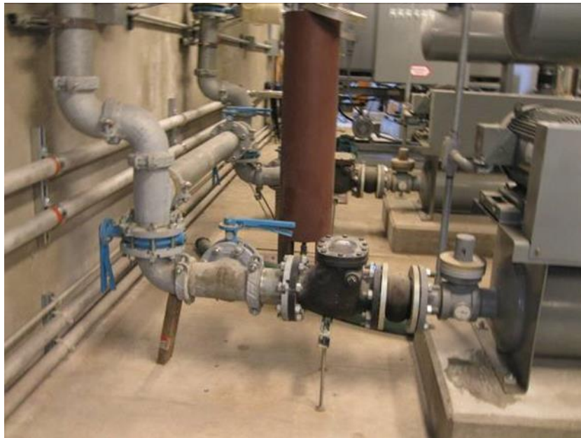
Figure 13–14. Rubber gate supply piping – note check valve
