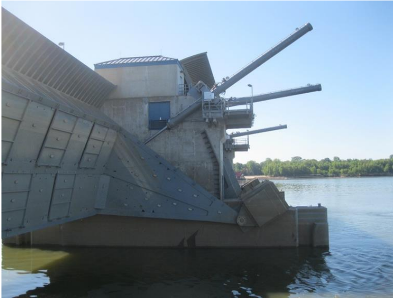
Figure 5–3. Olmsted Dam hydraulic, cylinder-operated tainter gates
