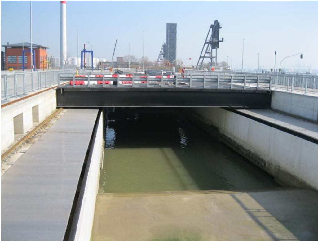
Figure 10–13. Wheelbarrow gate, Van Cauwelaert Lock, Antwerp, Belgium
