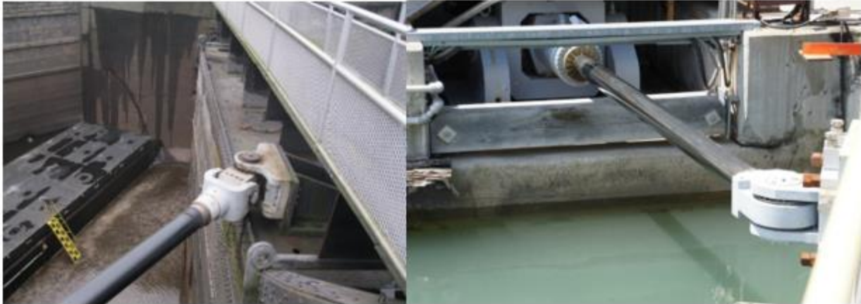
Figure 5–1. Miter gate ceramic-coated cylinder rod at Chittenden Lock, Seattle, and Welland Canal
