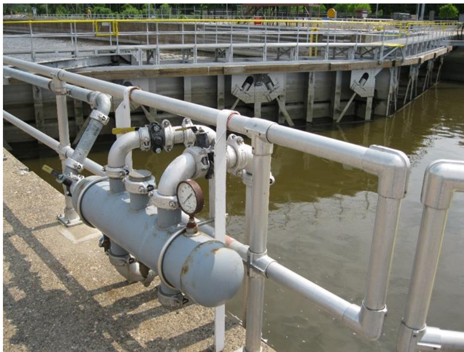
Figure 14–10. Typical diffuser supply system and manifold
