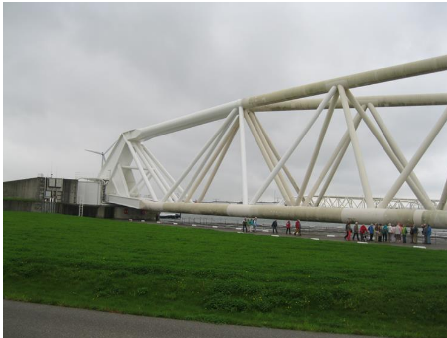
Figure 10–2. Maeslant Barrier sector gate arm and hinge
