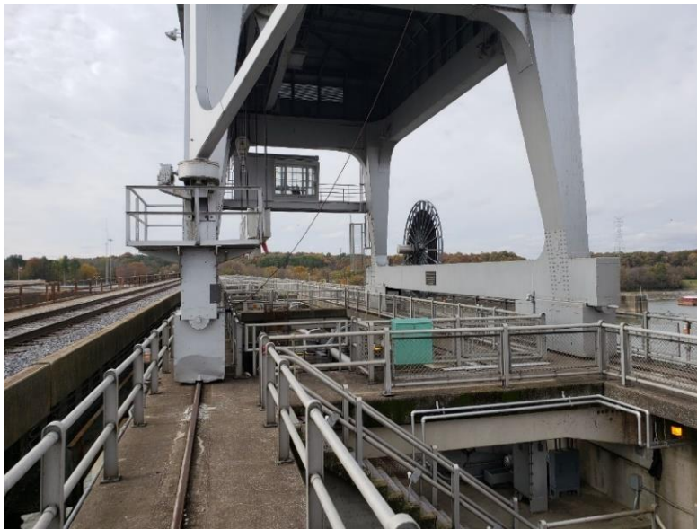
Figure 26-4. Barkley Project, electrical-powered reel for the powerplant intake/dam spillway crane
