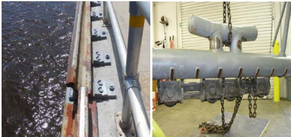
Figure 12–16. Lock and Dam 7 – rail misalignment and failure of towing bitt
