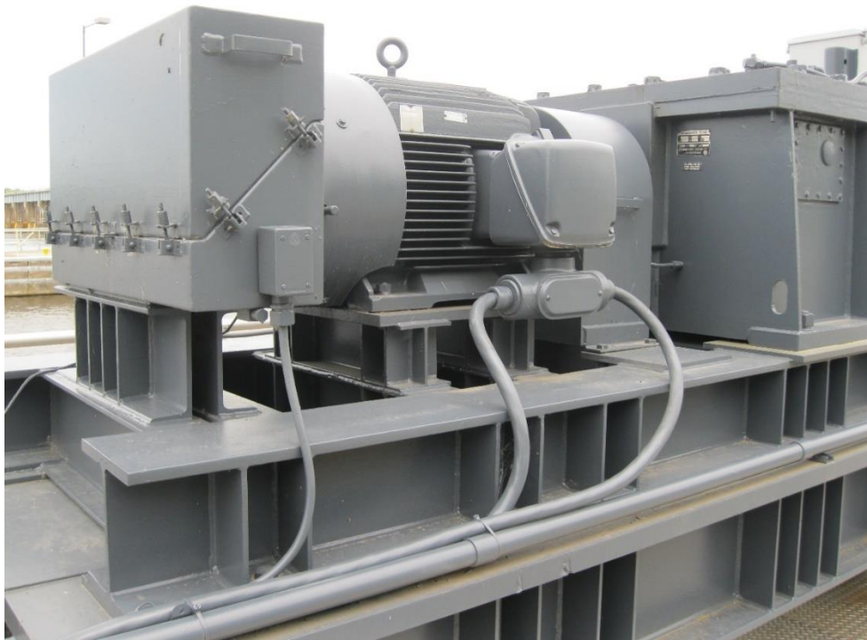
Figure 16–1. Miter gate drive motor, Lock 5, Mississippi River
