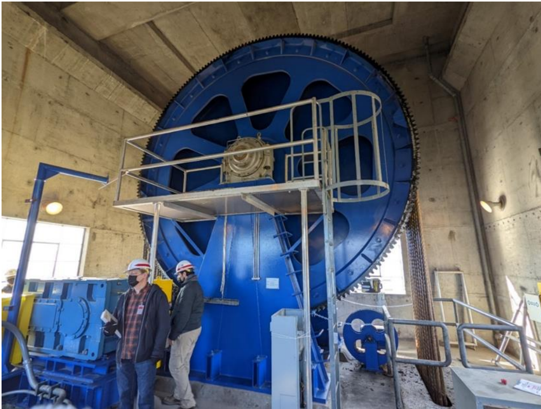
Figure 9–4. John Day downstream vertical gate friction sheave hoisting system
