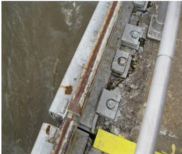
Figure 12-23. Too much gap in rail section of towing bitt
