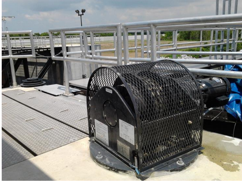
Figure 7–7. Backup winch system
