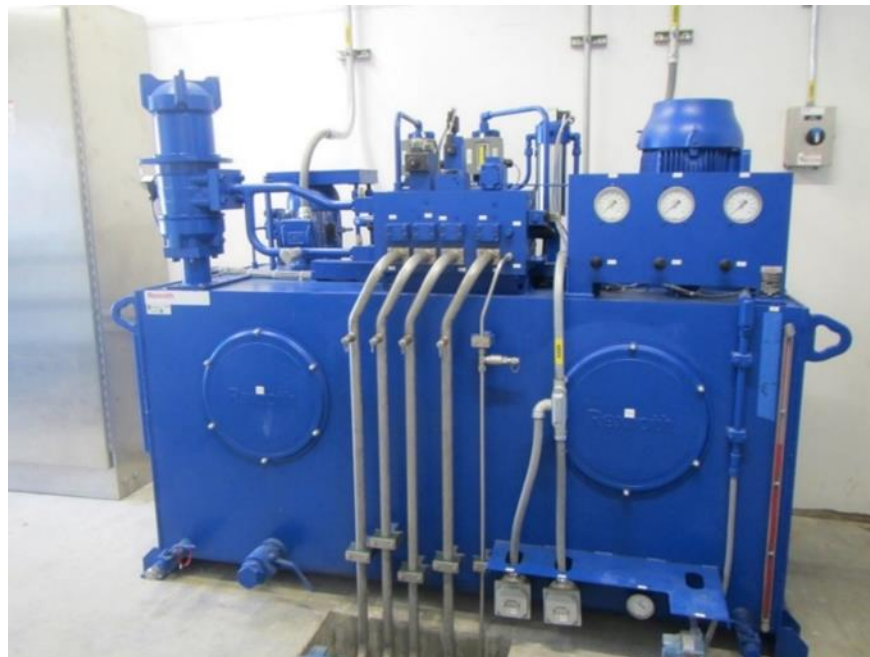
Figure 11–17. Olmsted Dam hydraulic power unit
