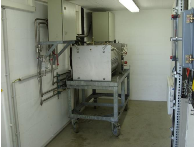
Figure 4–3. Compact hydraulic drive, Germany
