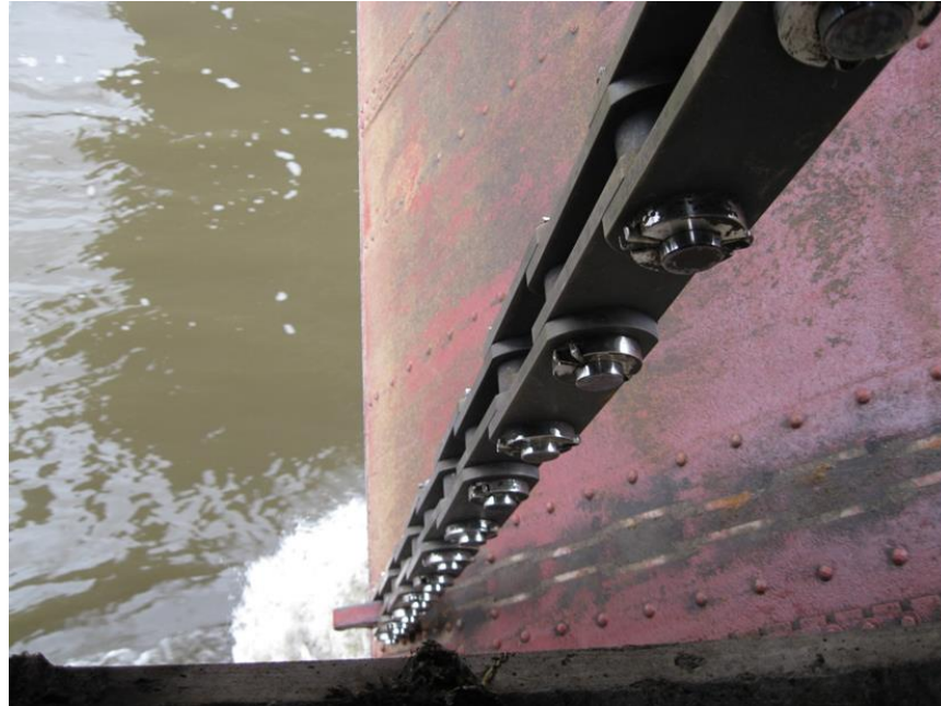
Figure 2–33. Engineered chain installation on a tainter gate
