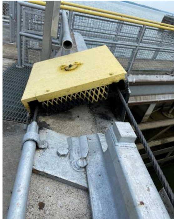
Figure 12–24. Old Hickory Lock – end sheave and towing bitt stop
