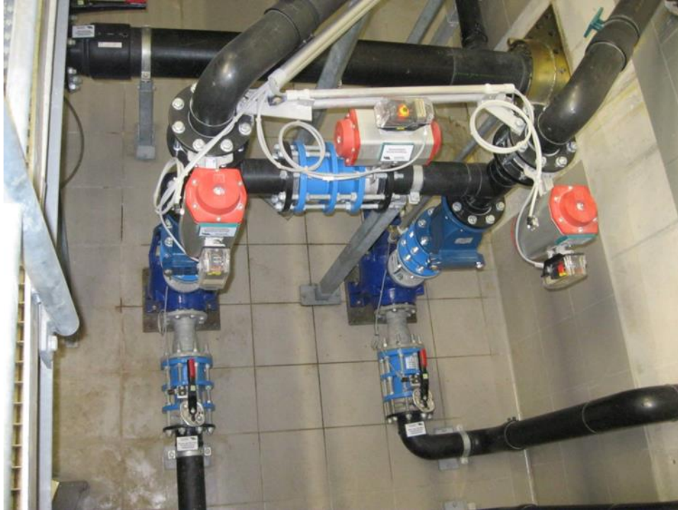
Figure 13–17. Water inflated gate – pumps and supply piping – Marklendorf Dam, Germany
