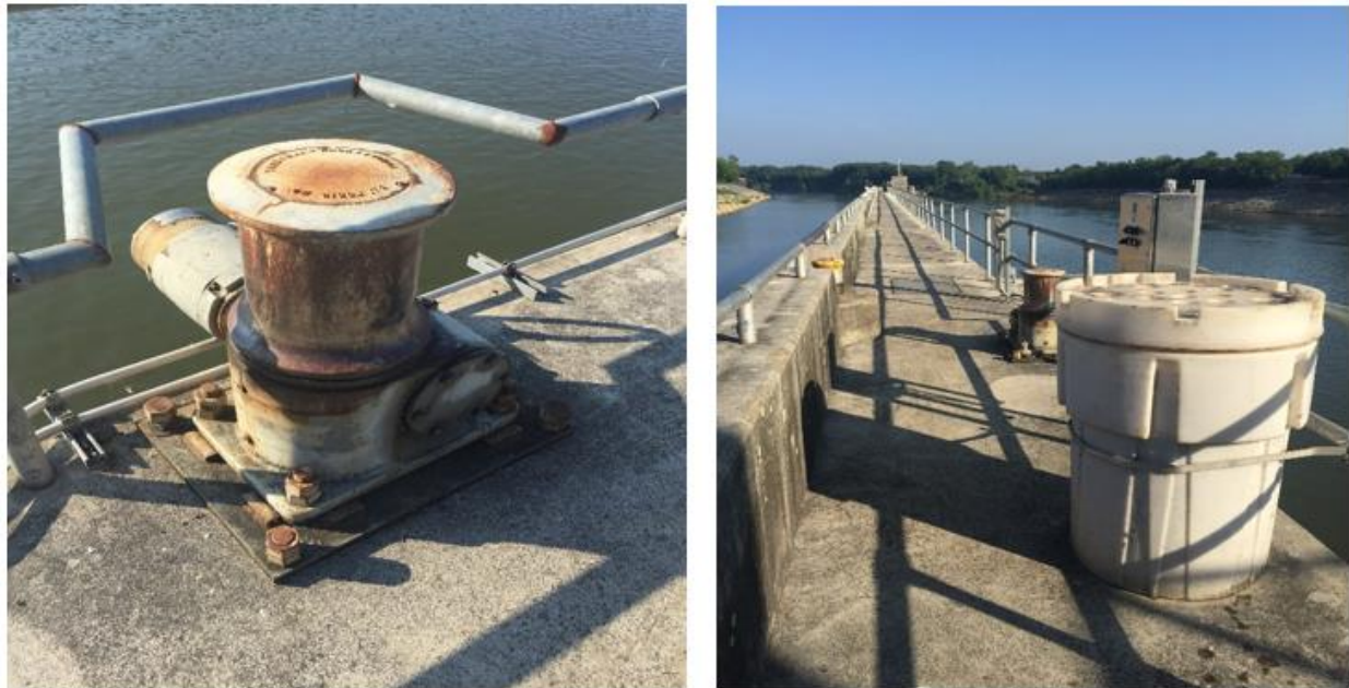
Figure 12–27. Old Hickory Lock – capstan
