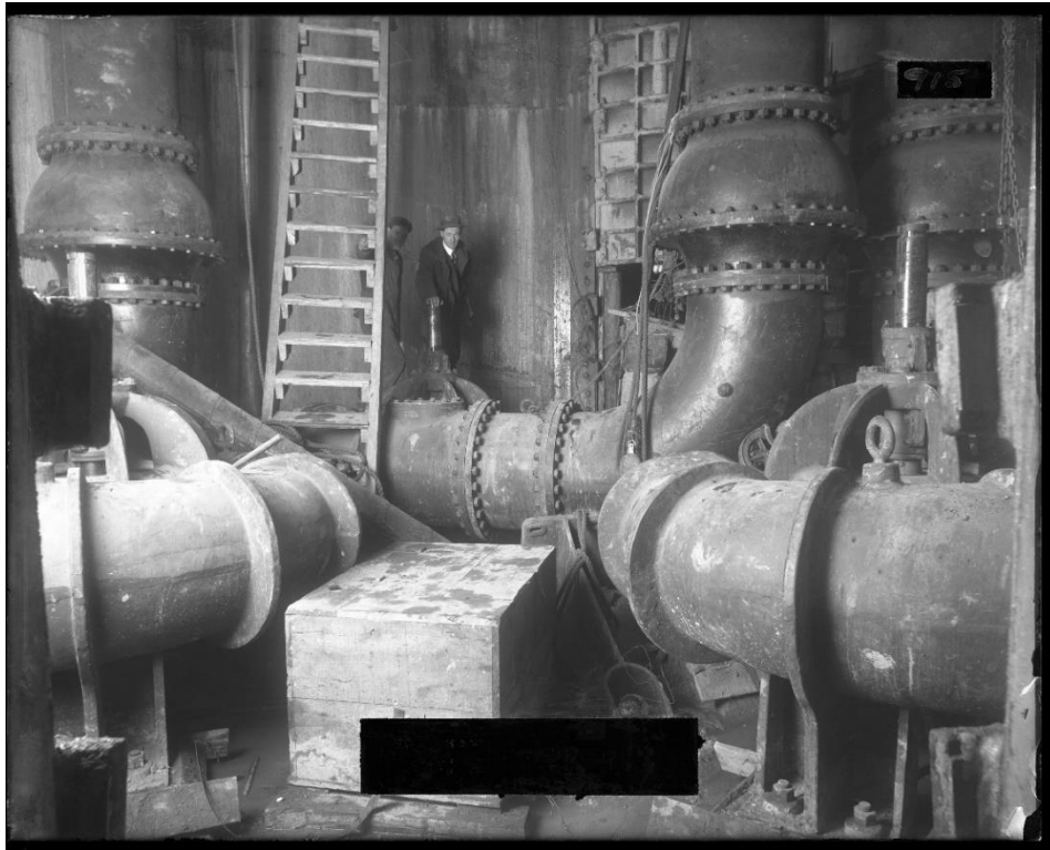
Figure 22–4. Davis Well double-suction centrifugal pumps from 1914
