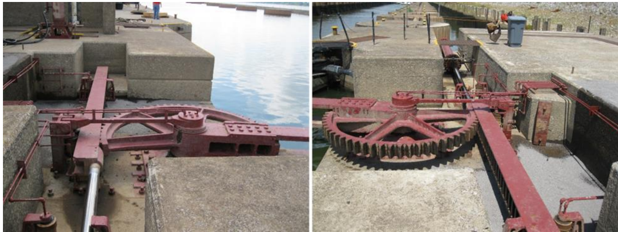
Figure 1–3. Hydraulic cylinder driving a rack and sector gear on Ohio River Locks
