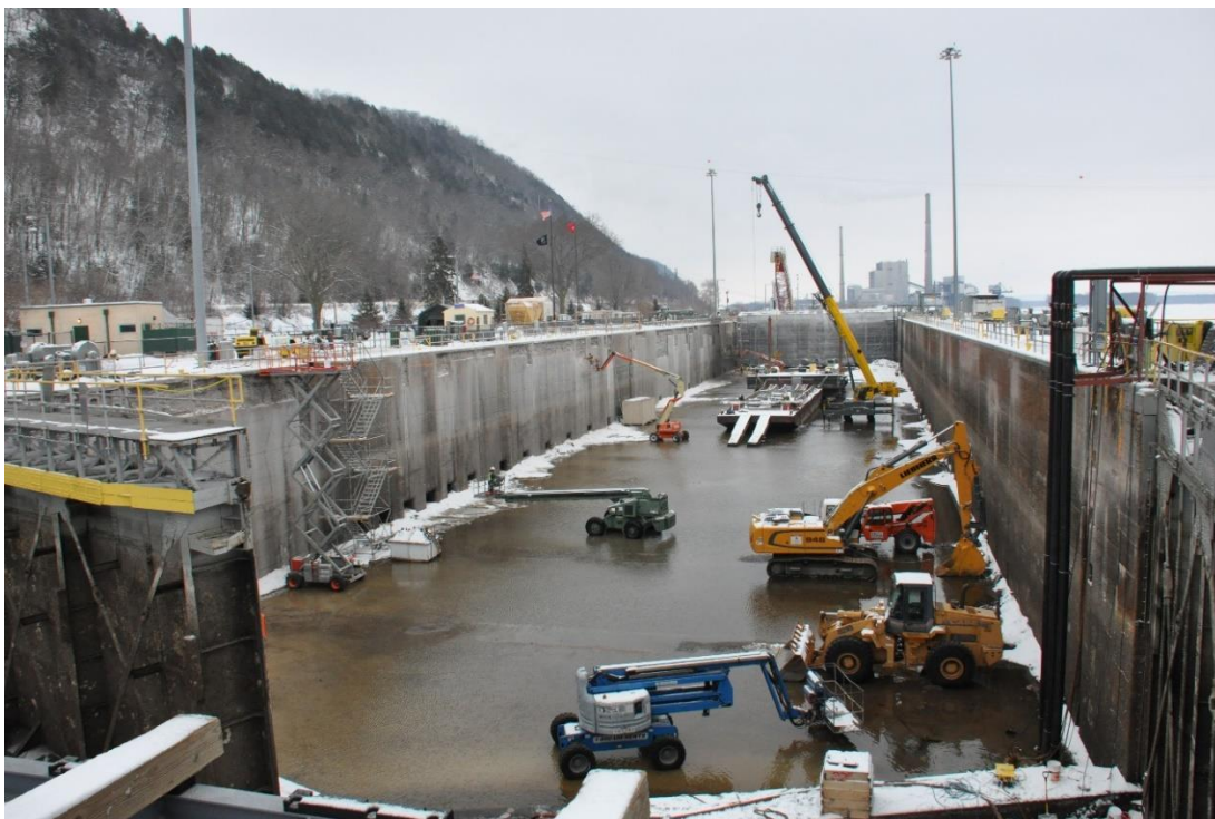
Figure 22–2. Lock 8 Mississippi River dewatering
