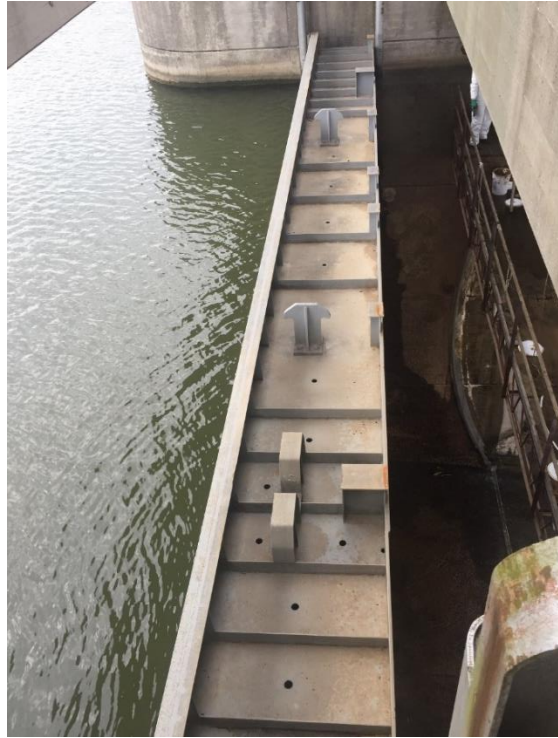
Figure 26–10. Old Hickory Dam, maintenance bulkheads for spillway gates
