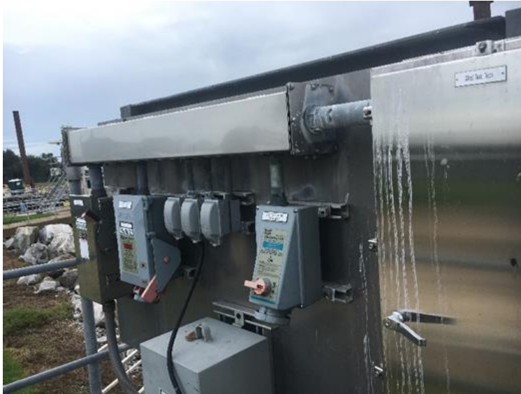
Figure 15–13. Example 2 – Shore power receptacles
