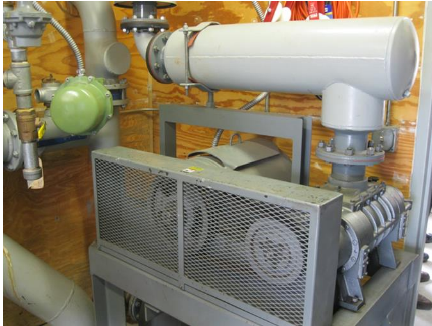
Figure 13–15. Air blower and receiver for rubber gate (Highgate Falls)
