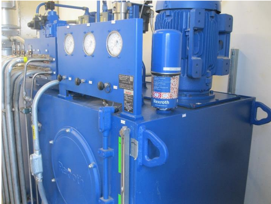
Figure 4–8. Olmsted Dam Hydraulic power unit and reservoir
