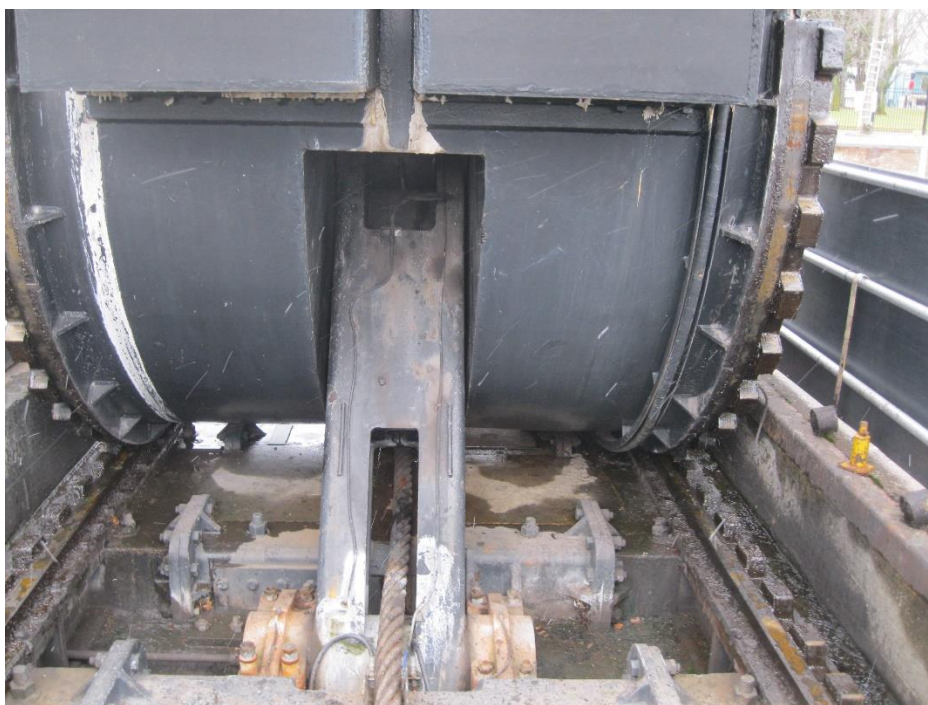
Figure 23-8. Poe Lock boom drive
