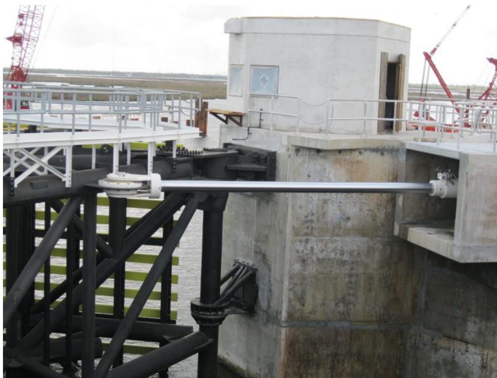
Figure 10–3. Inner Harbor Navigation Canal Sector gate, partially buoyant
