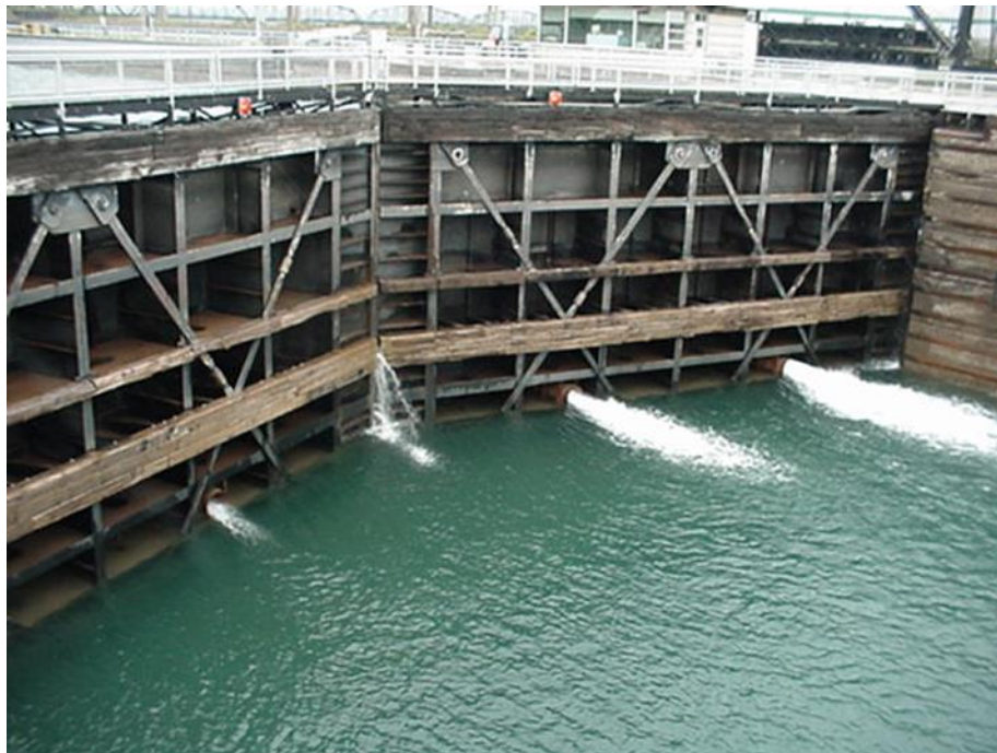
Figure 14–3. Soo Locks MacArthur Lock ice flushing valves
