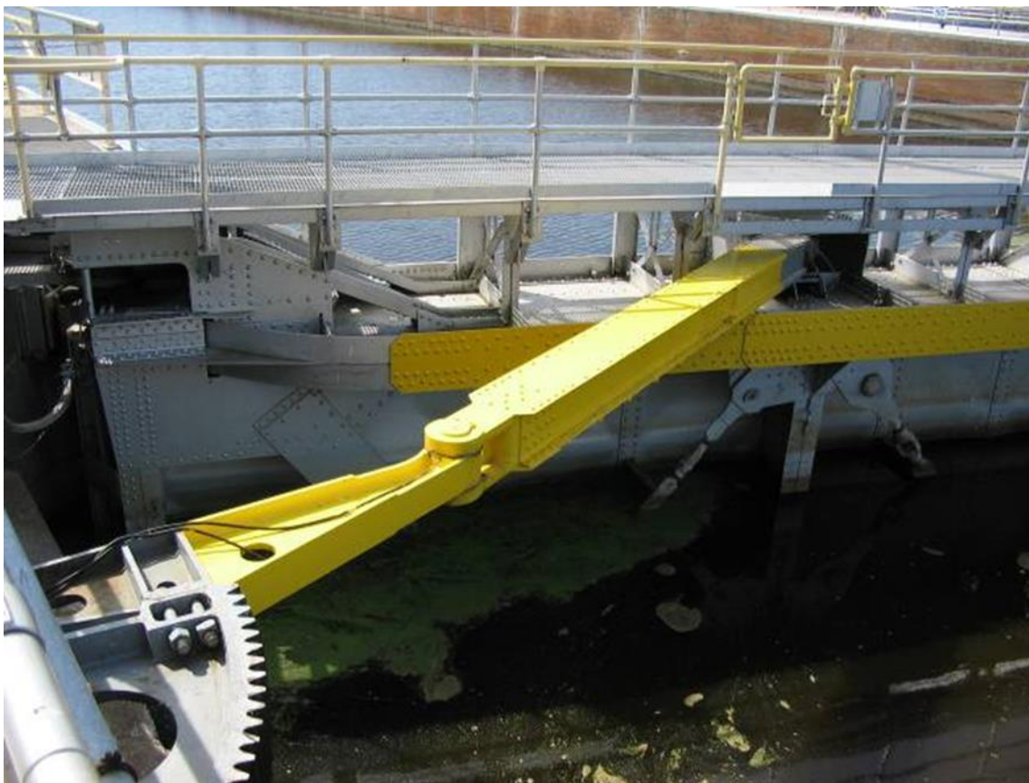
Figure 6–13. Miter gate strut arm
