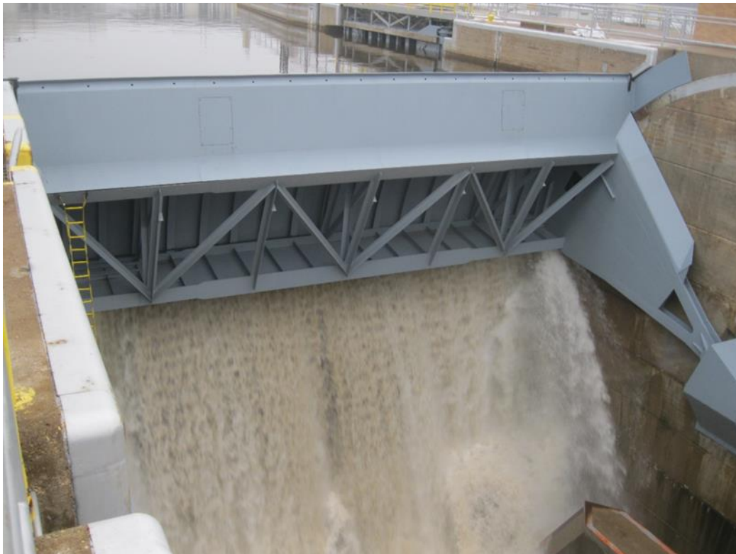
Figure 11–21. Upper St. Anthony Falls navigation lock submersible tainter gate
