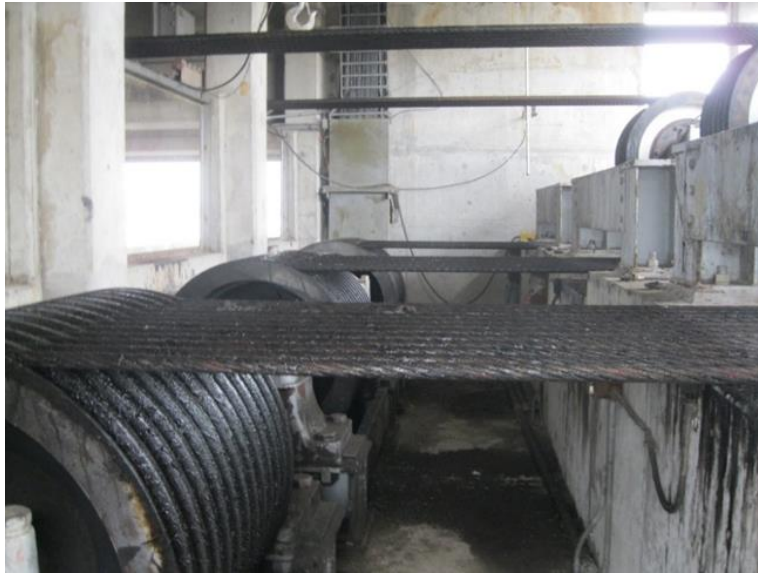
Figure 9-6. Mel Price Lock vertical gate wire rope lifting system
