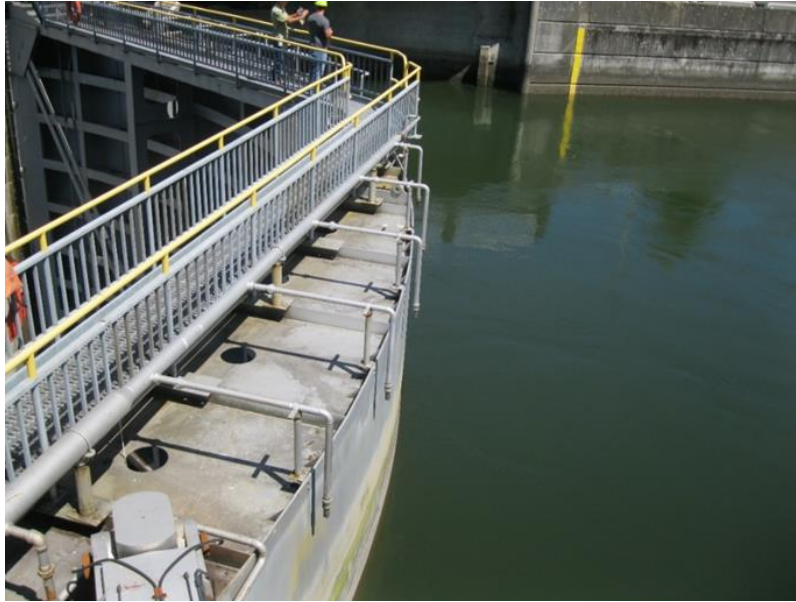
Figure 21–1. Miter gate spray system, Bonneville Lock
