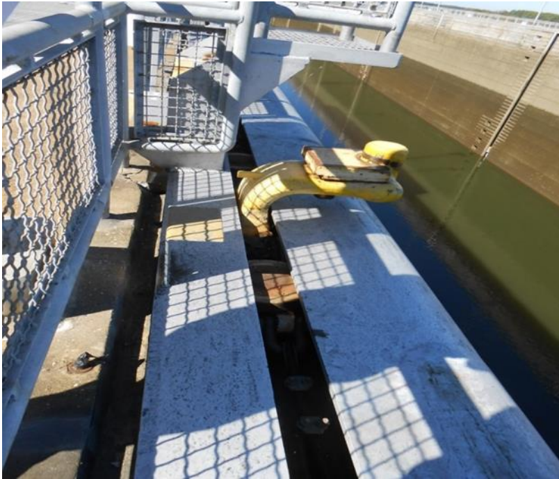
Figure 12-17. Pickwick main lock – towing bitt recess
