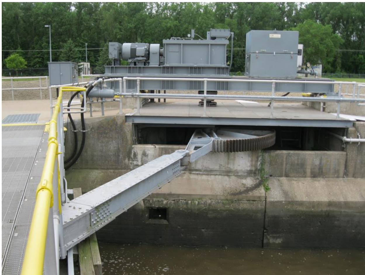
Figure 6-7. Modified Ohio River linkage with raised machinery
