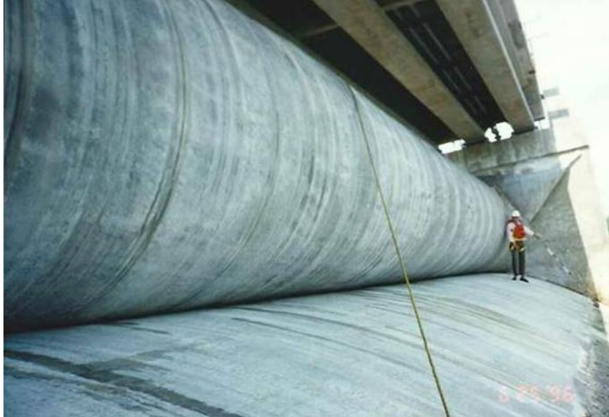
Figure 13–6. Coon Rapids rubber gate (Sumitomo) shown during an inspection of rubber bladder in 2006
