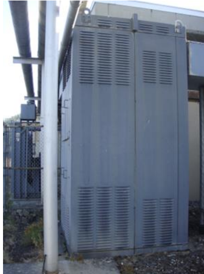
Figure 15–16. 480-volt current limiting reactor for 2-megavolt ampere service transformer
