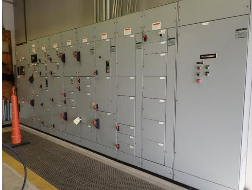
Figure 15–9. Low-voltage motor control center with programmable logic controller cabinet
