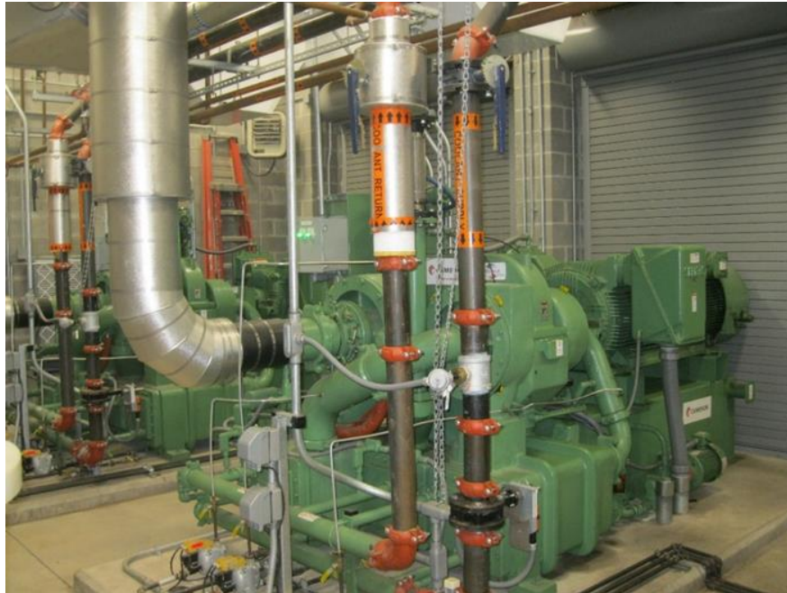
Figure 14–5. Soo Locks compressed air plant
