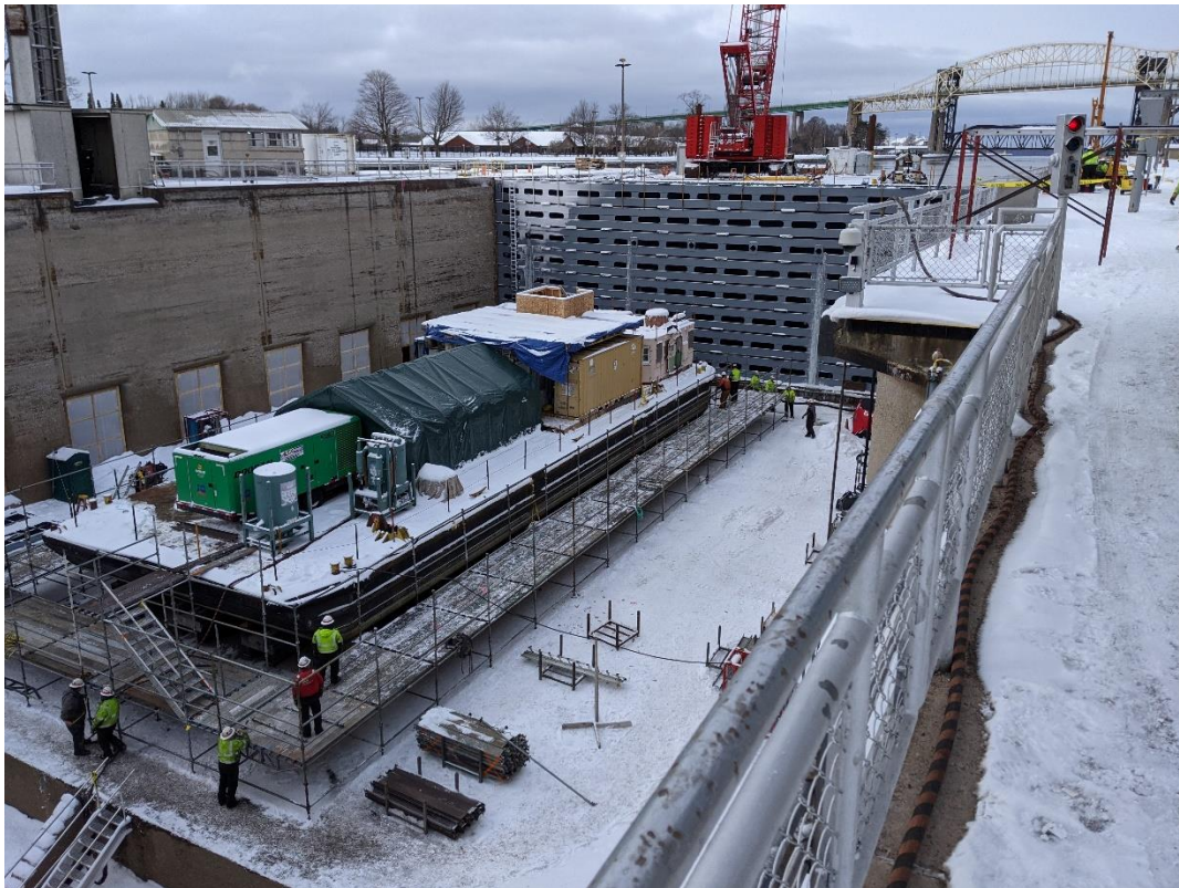
Figure 22–3. Soo Locks, Poe Lock dewatering
