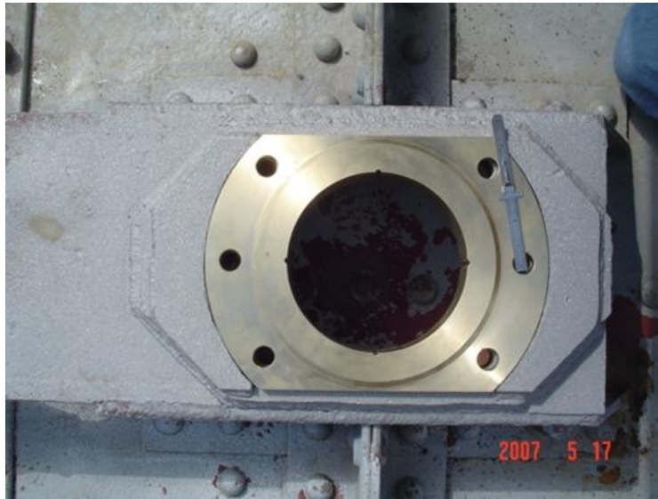
Figure 2–1. Plain bearing for a miter gate connection
