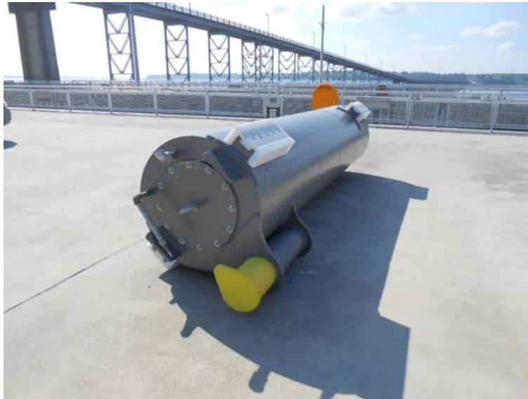
Figure 12–37. Wheeler main lock – single-post floating mooring bitt with ultra-high molecular weight polyethylene guides
