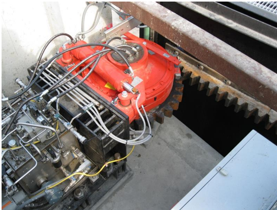
Figure 7–2. Hydraulically operated pinion gear and rack
