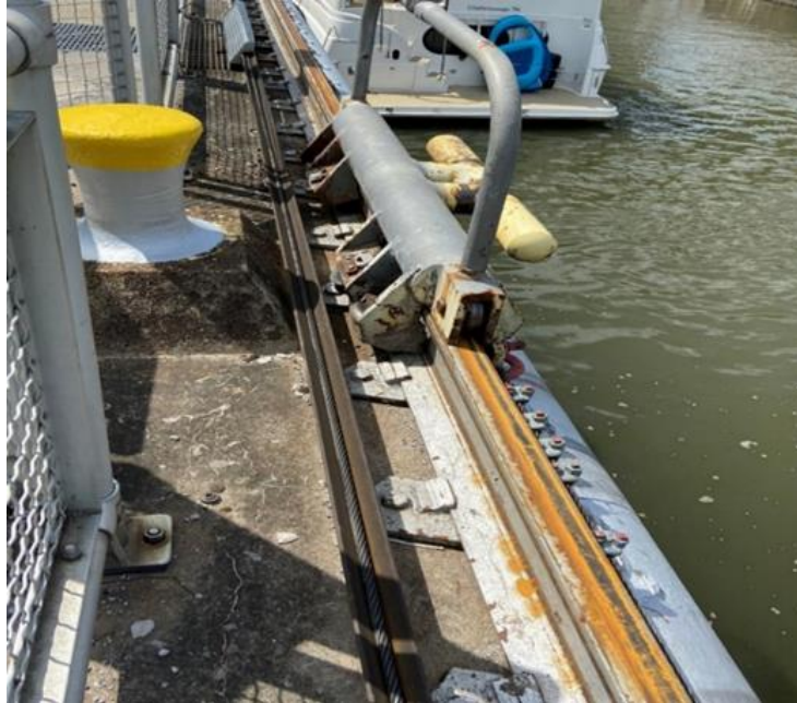
Figure 12–20. Existing Chickamauga Lock – rail located at top of the lock wall; towing bitt with horn assembly at 0 degree with the horizontal plane
