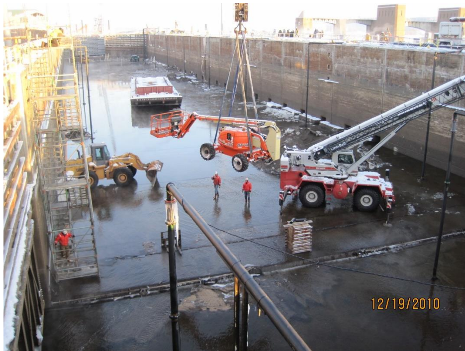
Figure 22–1. Lock 10 Mississippi River dewatering
