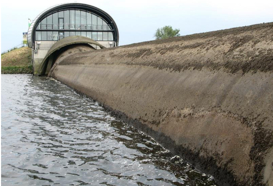
Figure 13–7. Ramspol Storm Surge Barrier rubber gates, Netherlands, test closure photos Rijkswaterstaat
