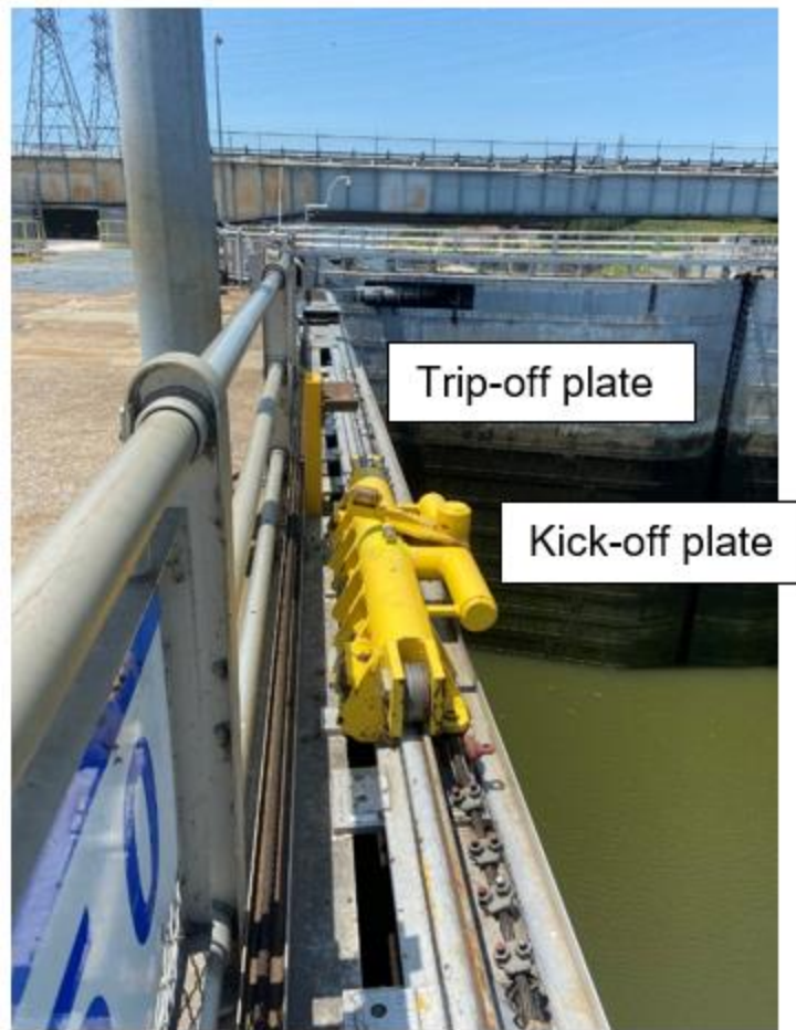
Figure 12–29. Existing Kentucky Lock – towing bitt kick-off plate and trip-off plate
