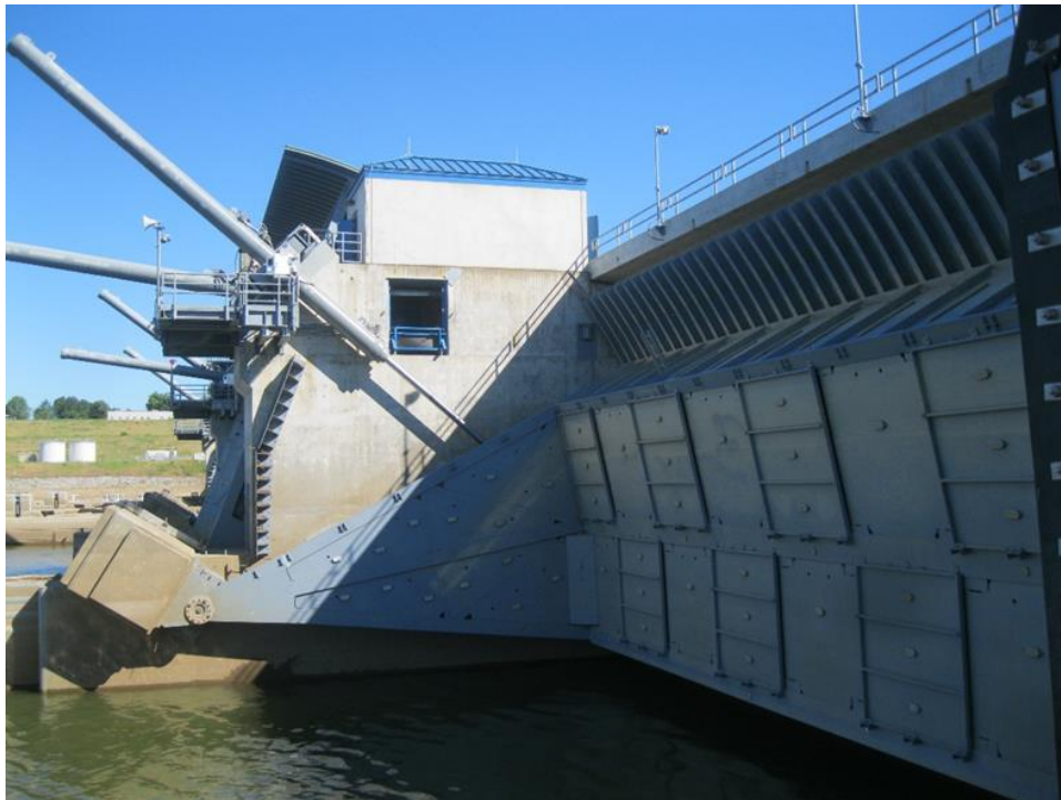
Figure 11–16. Olmsted Dam hydraulic-driven tainter gates
