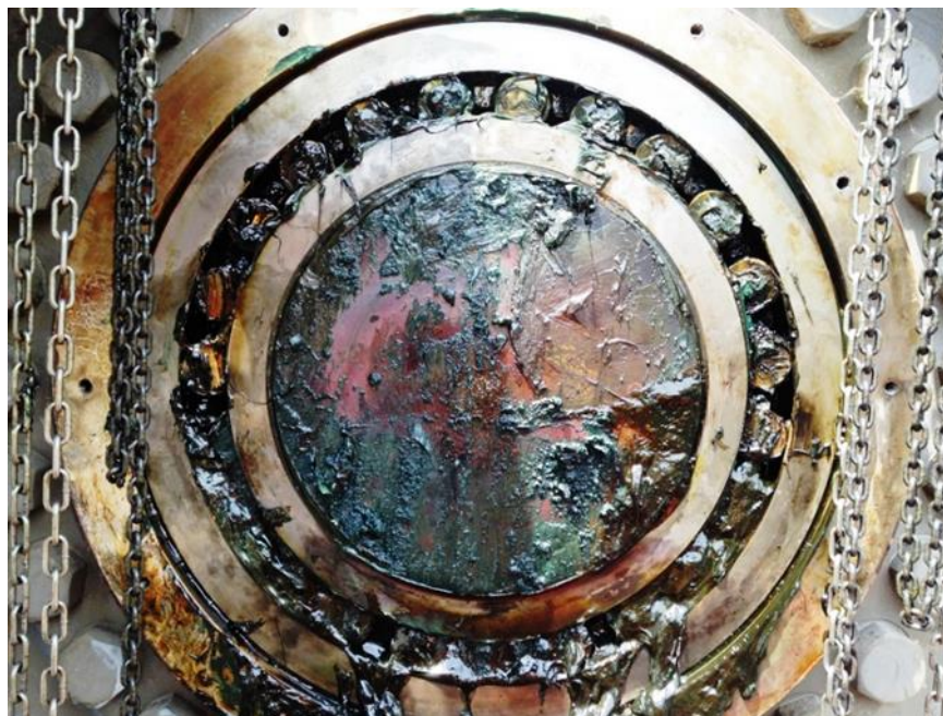
Figure 11–11. Spherical bearing for Whittier Dam gate
