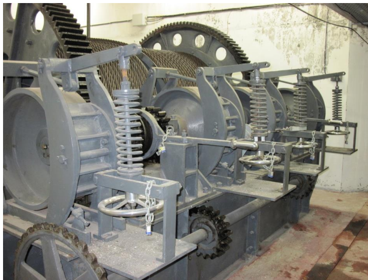
Figure 23–11. Brake drum at St. Lambert Lock, Maisonneuve Region
