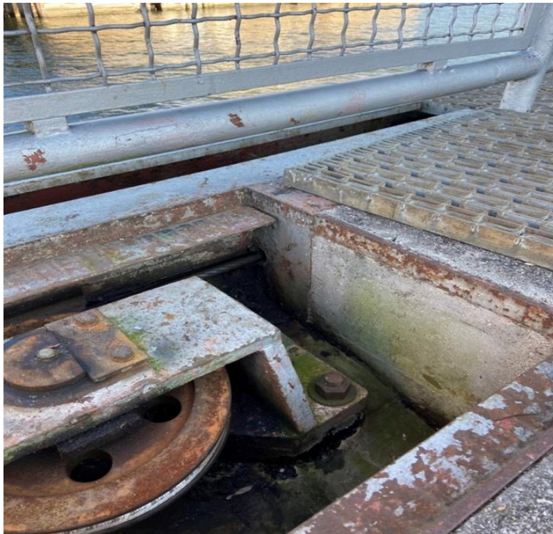
Figure 12-18. Pickwick main Lock – wire rope in embedded concrete
