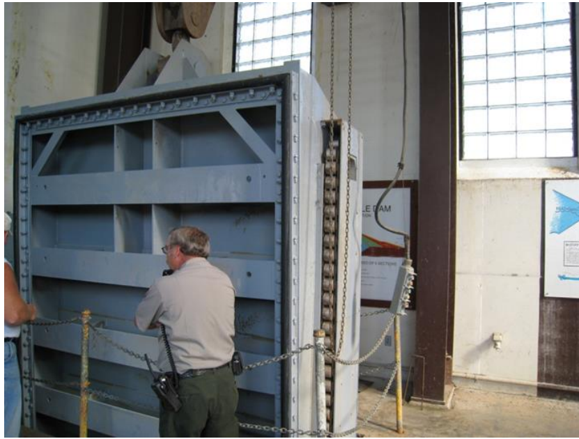
Figure 9–15. Tractor-style gate
