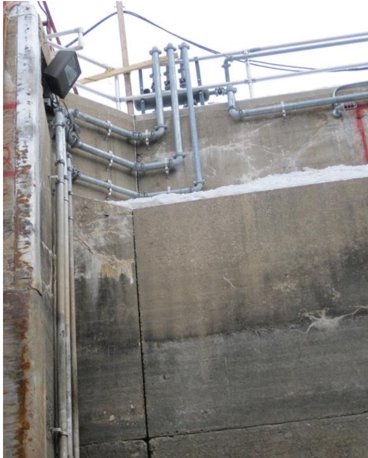
Figure 14–12. Bubbler piping attachment using offset clamps
