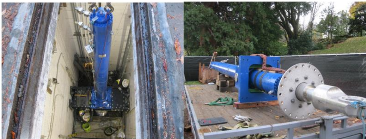
Figure 5–9. Chittenden Lock culvert valve cylinder
