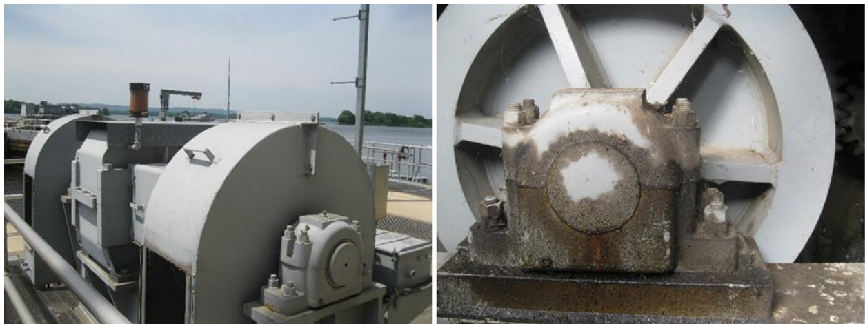
Figure 2-5. Pillow block bearings for culvert valve machinery
