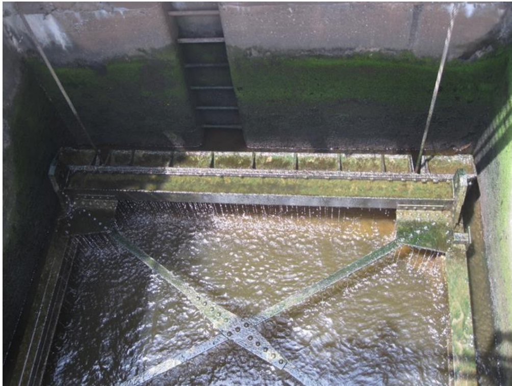
Figure 8-5. Lock 4, Mississippi River culvert tainter valve showing wire rope connections
