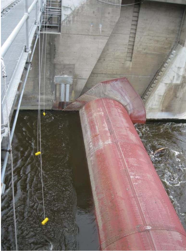
Figure 11-29. Roller gate detail
