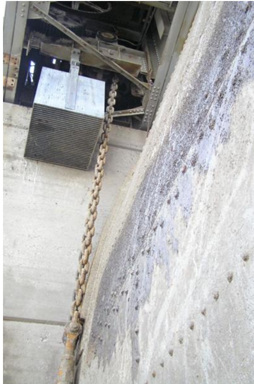
Figure 2–26. Pocket wheel chain hoist with chain locker
