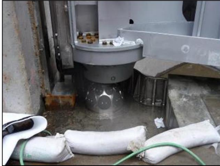
Figure 3–8. Miter gate pintle at The Dalles Lock
