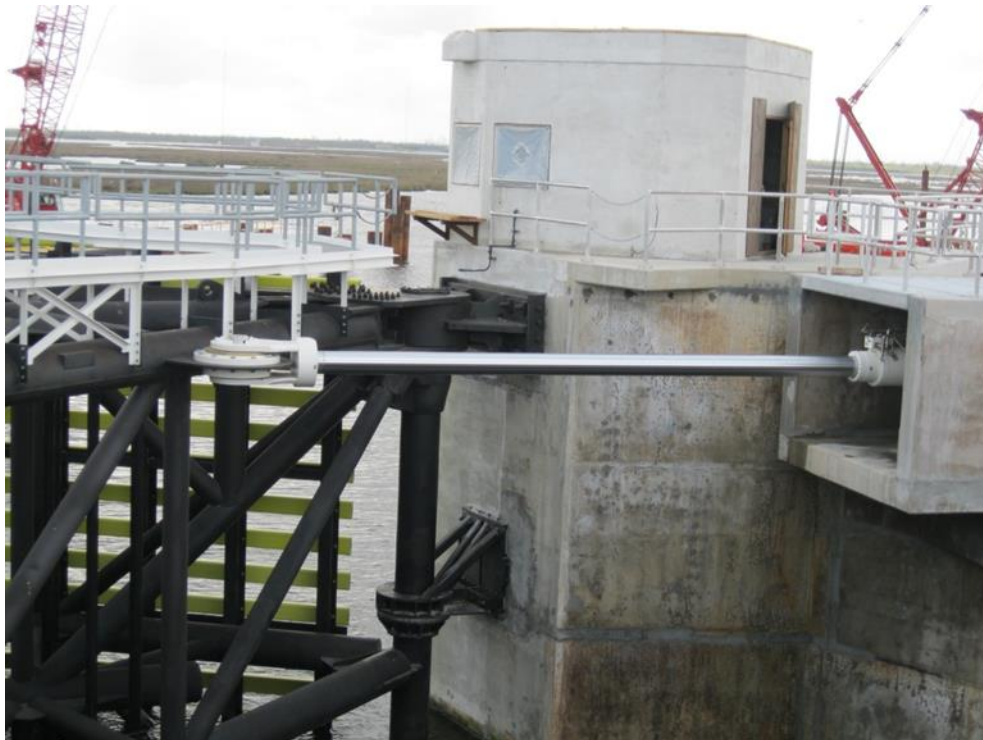
Figure 7–3. Hydraulic cylinder-driven sector gate, New Orleans Inner Harbor Navigation Canal
