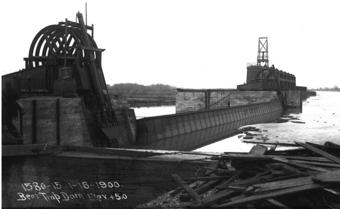
Figure 10–25. Bear trap gate in the Ohio River
