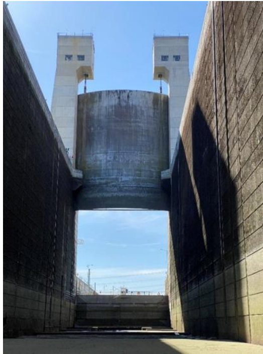
Figure 9–3. Vertical downstream overhead gate John Day Lock
