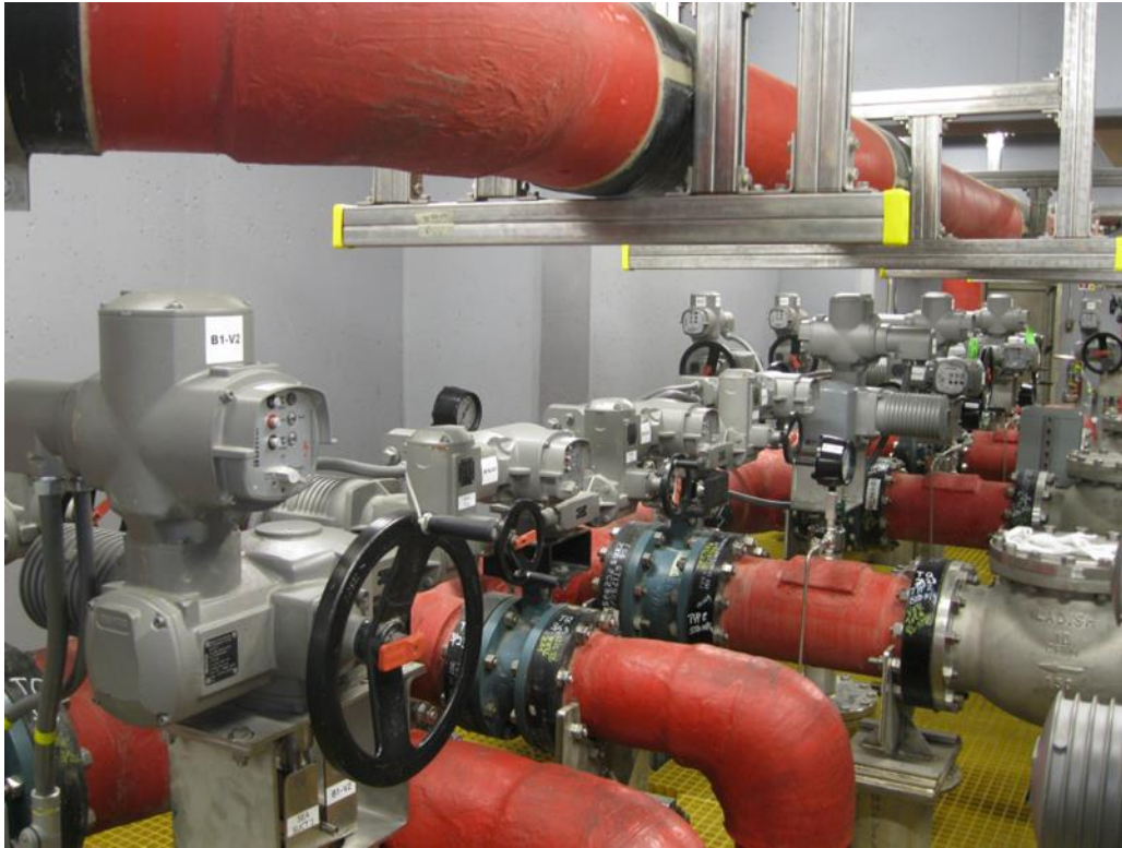
Figure 10–7. Pumping system for Inner Harbor Navigation Canal barge gate
