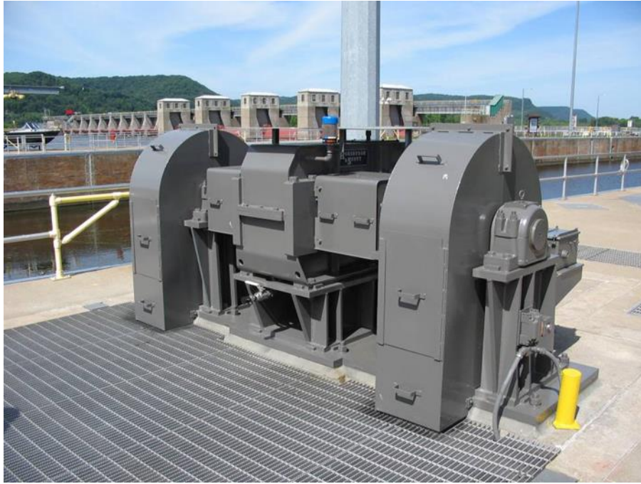
Figure 8-6. Electric motor-driven tainter valve hoist
