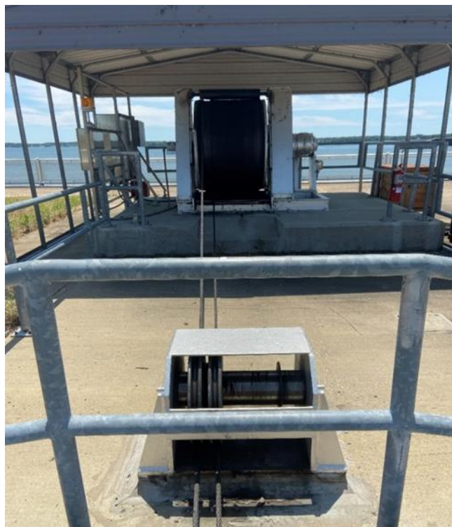
Figure 12-4. Existing Kentucky Lock – sliding sheave
