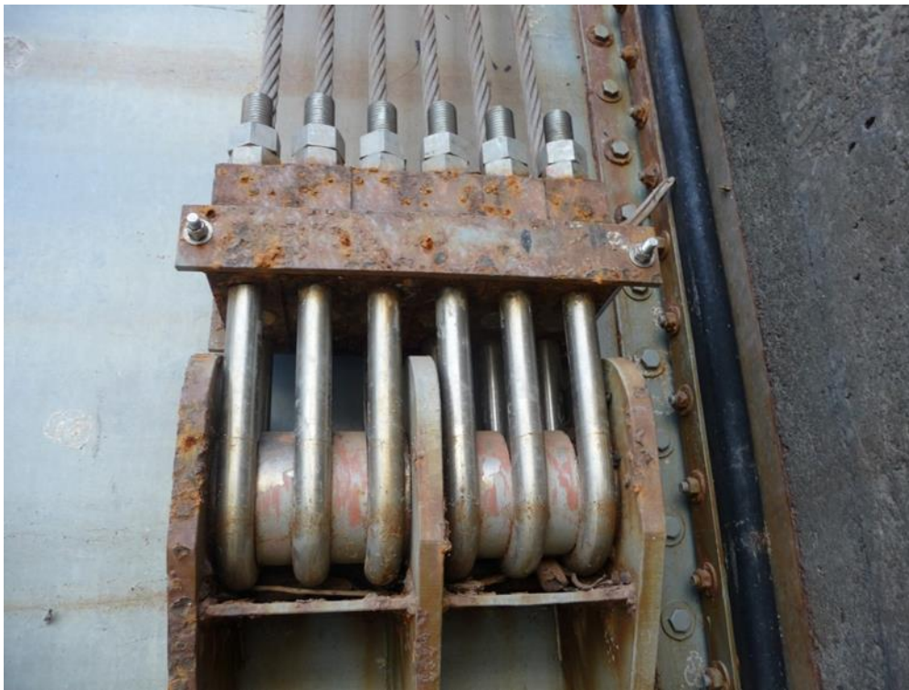
Figure 2–39. Multiple wire rope and gate connection detail for tainter gate lifting application
