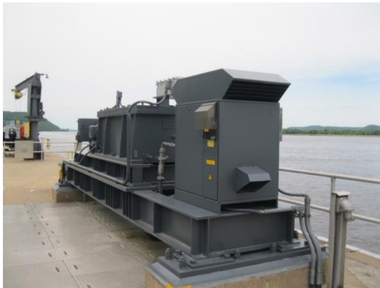
Figure 14–6. Air compressor installed on lock miter gate machinery platform
