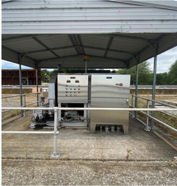
Figure 12–30. Barkley Lock – tow haulage control at winch unit
