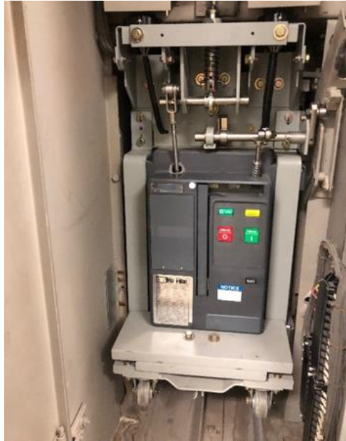
Figure 15–11. 5-kV 1,200-amp vacuum circuit breaker
