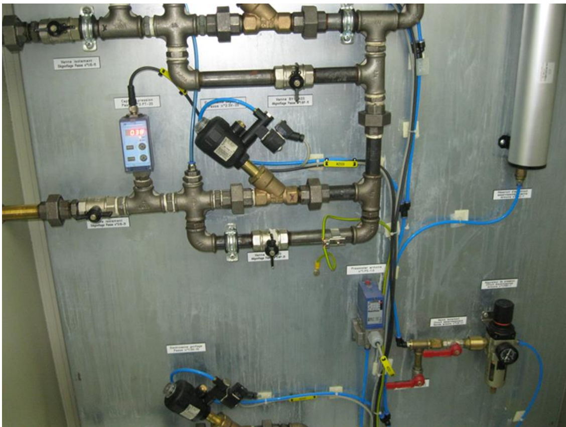
Figure 13–20. Pneumatic control system – Auxonne Dam
