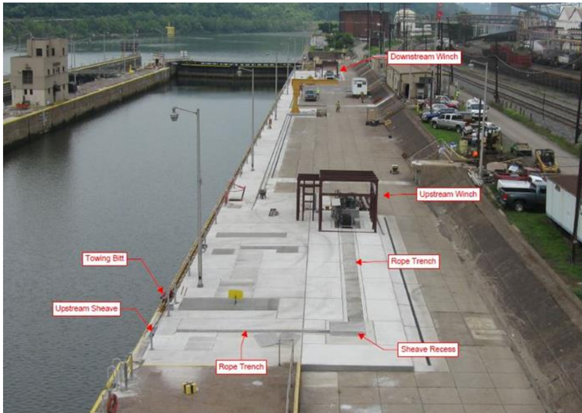
Figure 12-9. Braddock Lock – torque-control tow haulage layout
