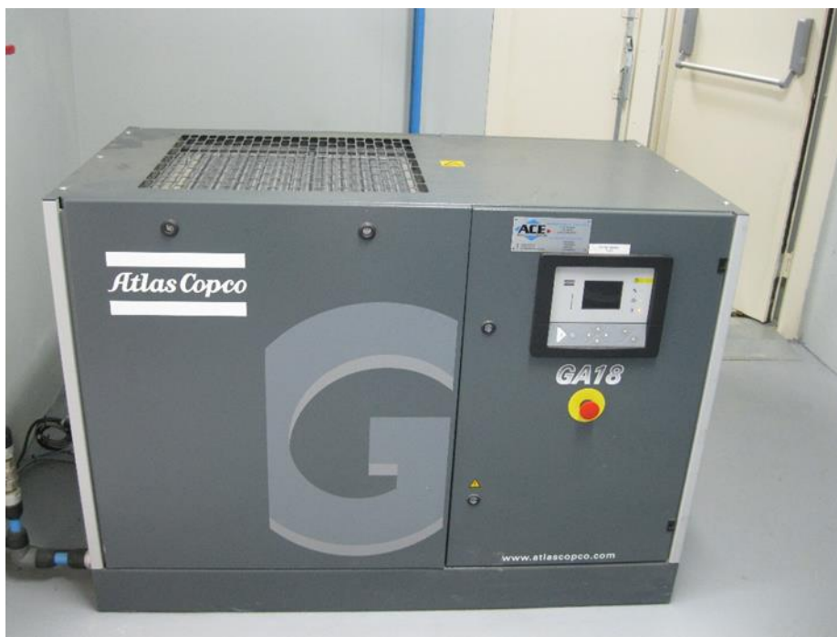
Figure 13–16. Rotary screw compressor, Auxonne Dam
