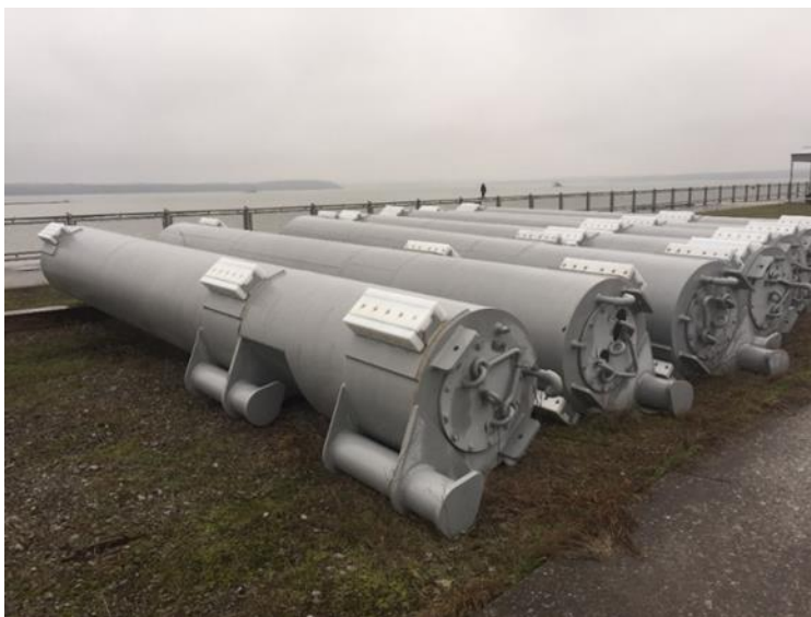
Figure 12-35. Barkley Lock – double-post floating mooring bitt with ultra-high molecular weight polyethylene guides (new design)
