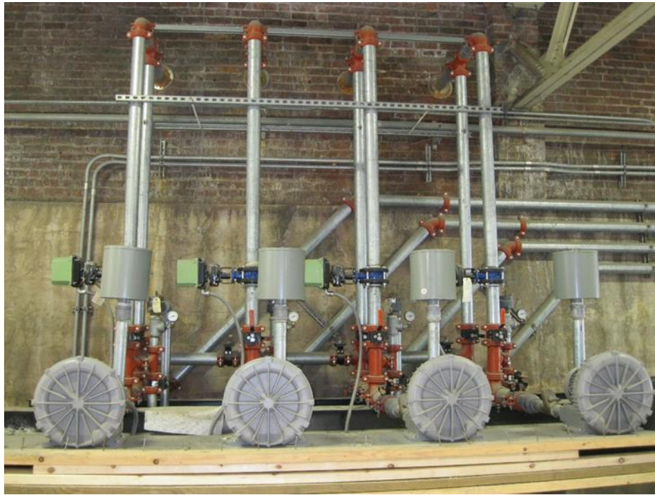
Figure 13–13. Rubber gate air blowers, supply piping, and manifold – Curtis Dam
