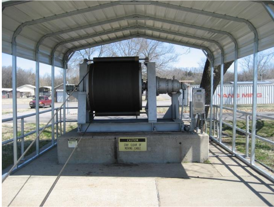
Figure 12–6. Cheatham Lock – new single winch unit with planetary gearbox
