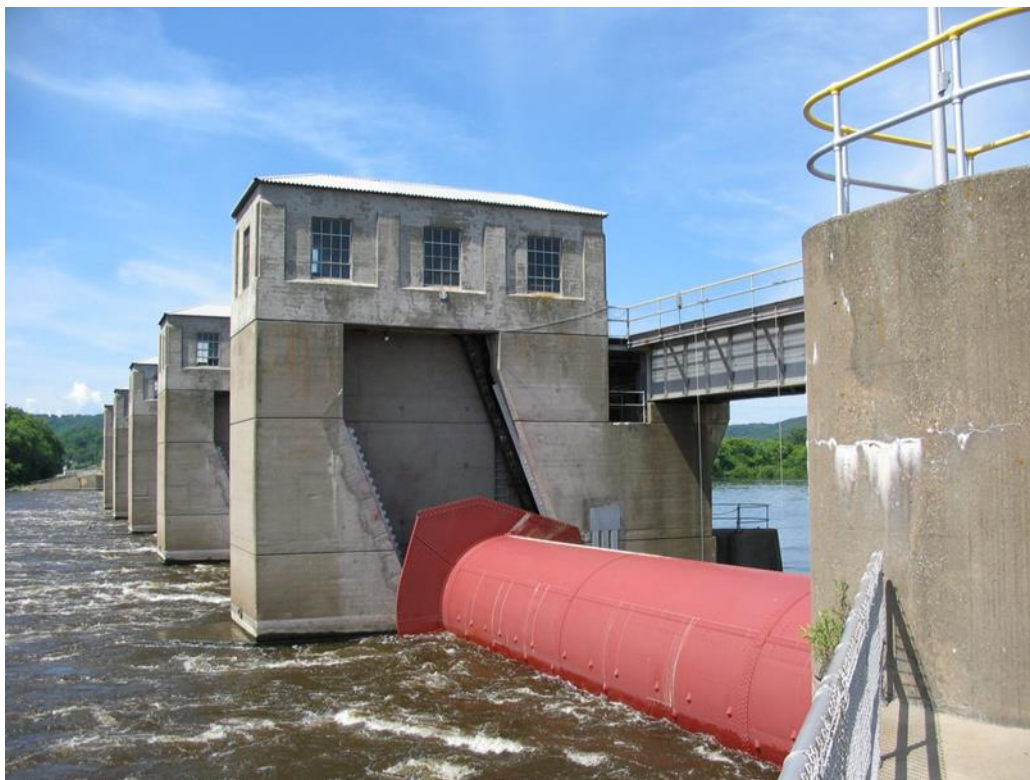
Figure 11–26. Roller gate, Mississippi River
