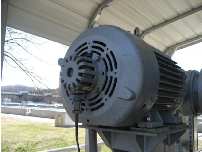
Figure 12–8. Cheatham Lock – encoder and electric motor
