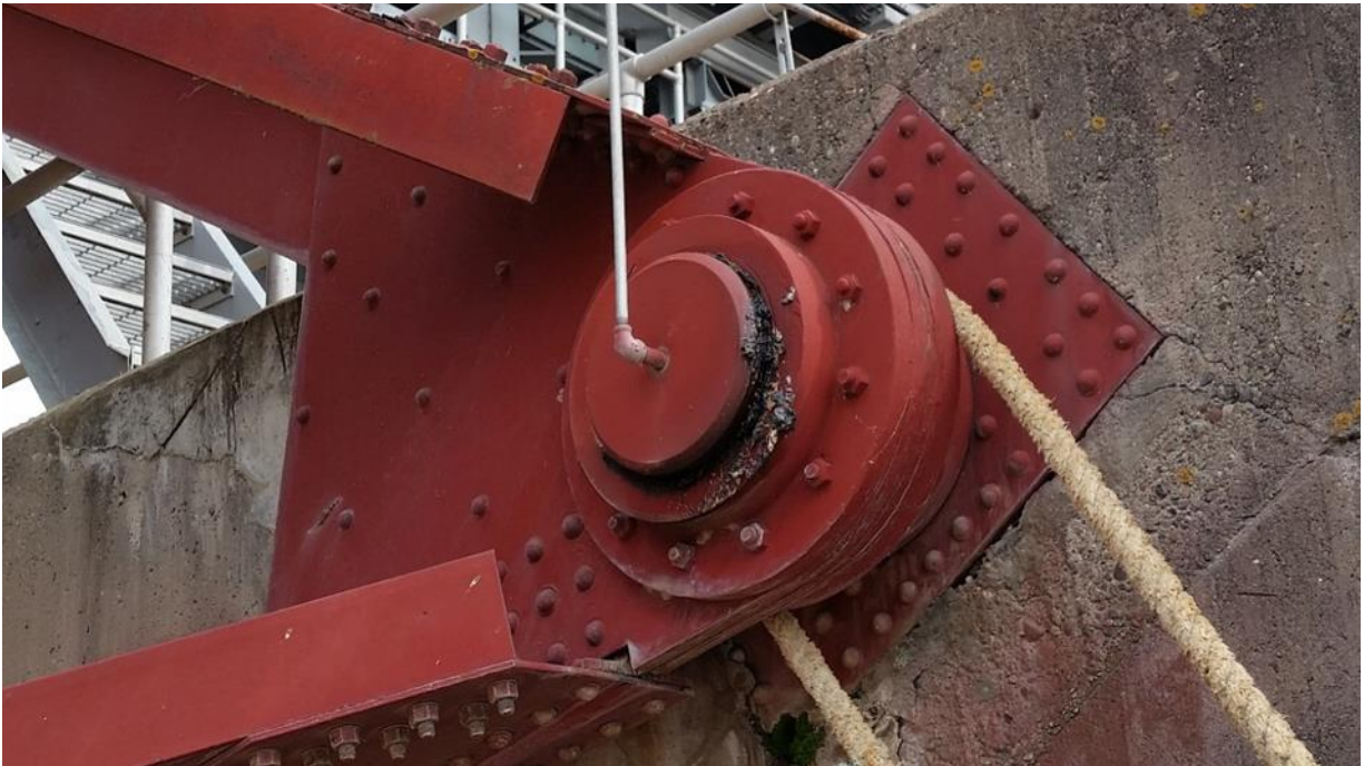
Figure 11–9. Tainter gate trunnion bearing
