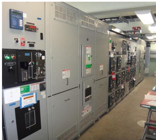
Figure 15–10. Low-voltage double-ended switchgear with power circuit breakers
