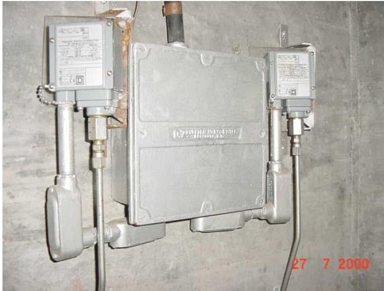
Figure 2–18. Hydraulic pressure limit switch
