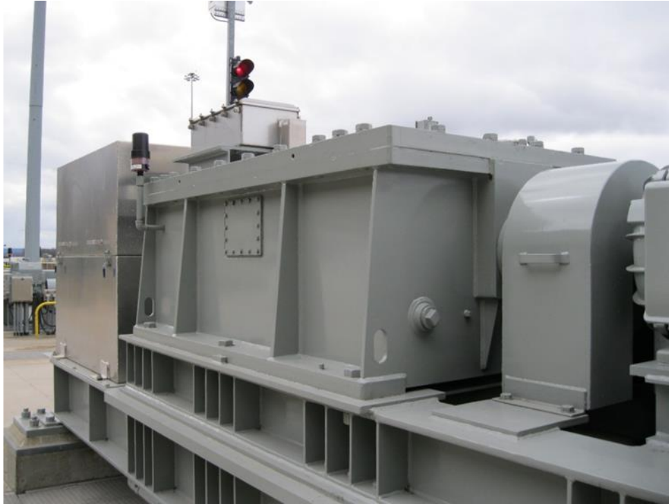
Figure 2–38. Miter gate speed reducer
