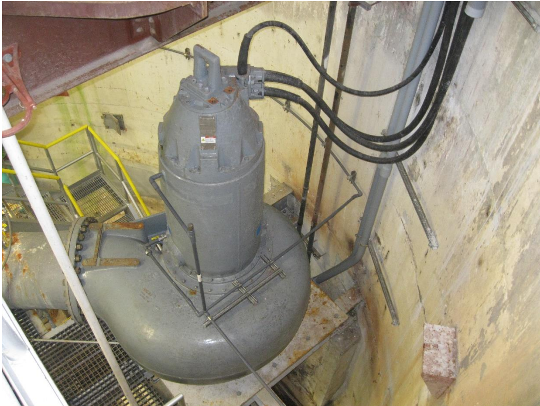
Figure 22–9. New pumps for Chittenden pumping plant 2016
