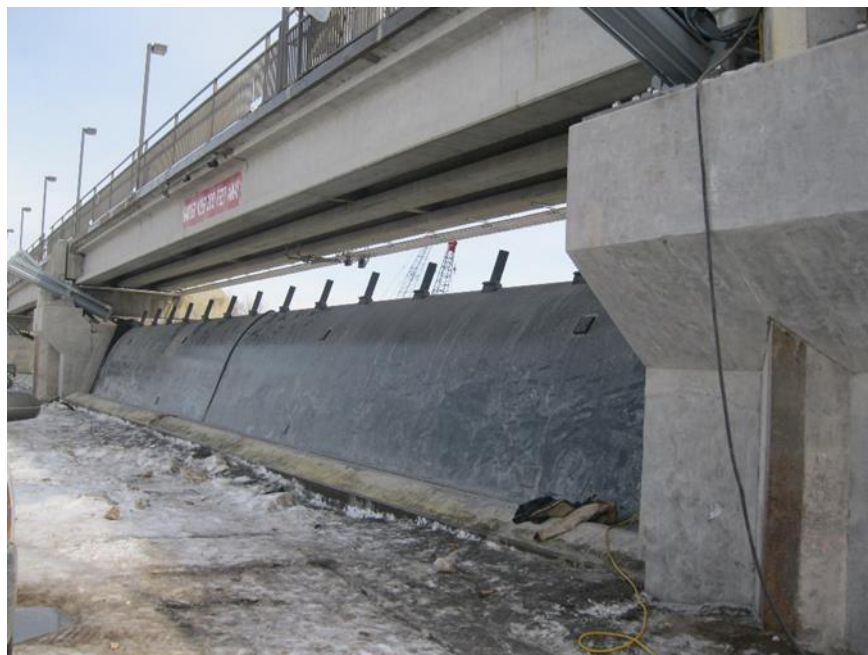
Figure 11-23. Coon Rapids Dam hinged crest gate (dewatered condition)
