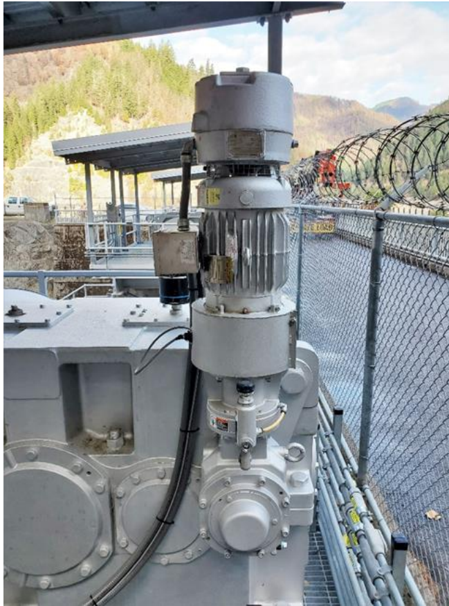
Figure 2–10. Motor-mounted disc brake
