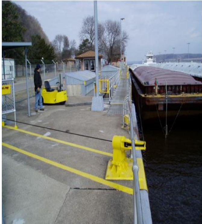
Figure 12–11. Typical tow haulage with fairlead on the Upper Mississippi River
