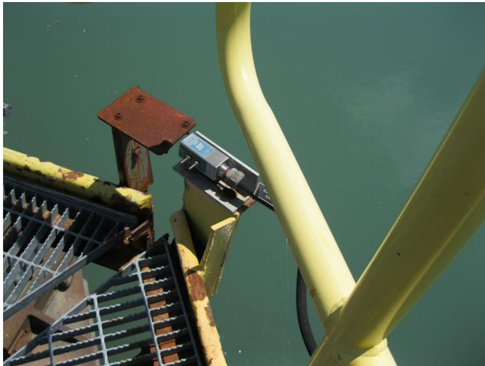
Figure 6–17. Miter gate position limit switch
