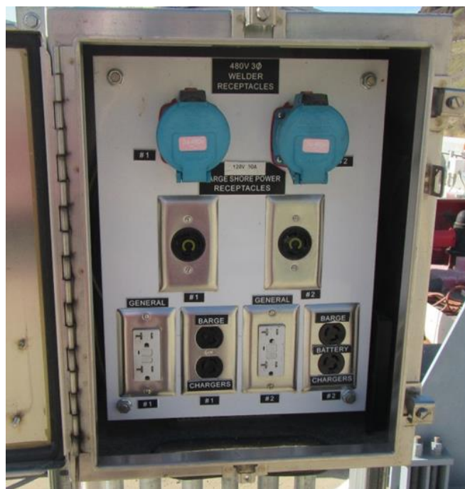
Figure 15–12. Example 1 – Shore power receptacles
