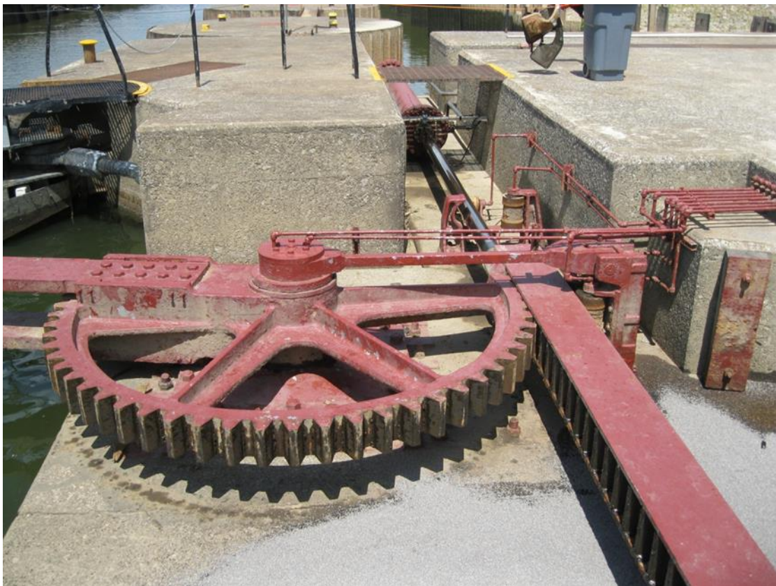
Figure 6–5. Lock 52, Ohio River, traditional Ohio linkage with toothed rack gear
