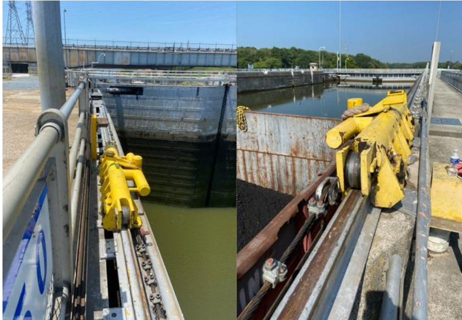
Figure 12-14. Existing Kentucky Lock and Old Hickory Lock – towing bitt with kick-off plate and trip-off plate
