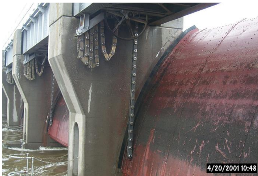
Figure 11-14. Hoist chain gate connection
