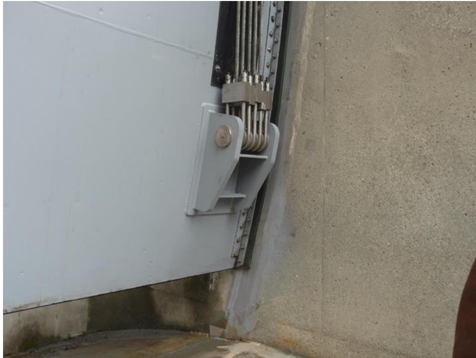
Figure 11–13. Wire rope gate connection
