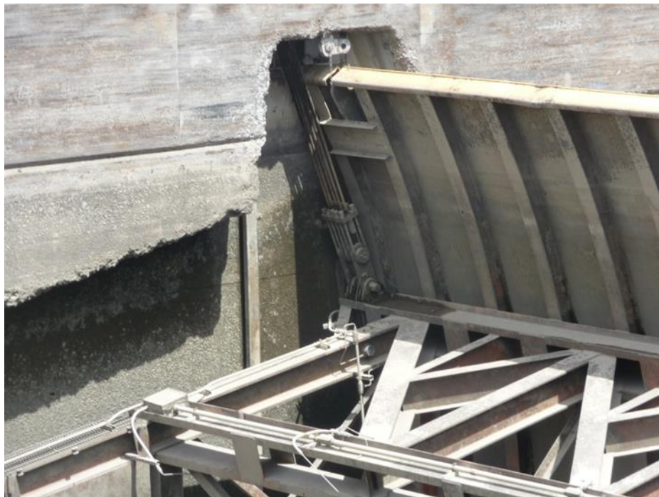
Figure 11–20. Common gate connection style and location for submersible tainter gates
