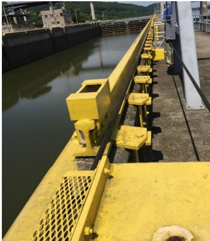
Figure 12–21. Murray Lock – rail located at top of the parapet wall
