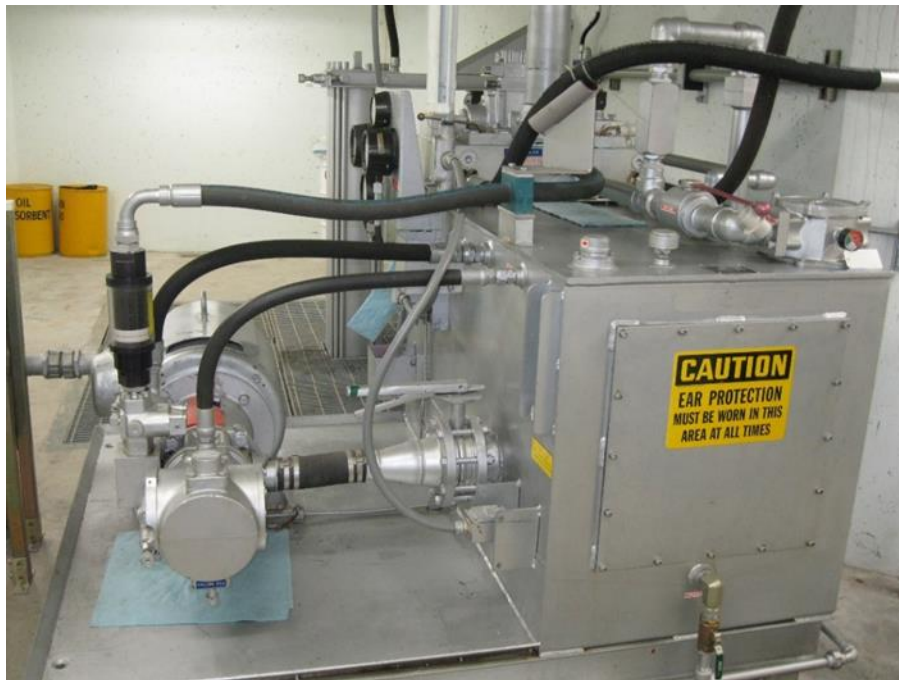
Figure 4–1. Tainter valve hydraulic power unit at Bonneville Lock
