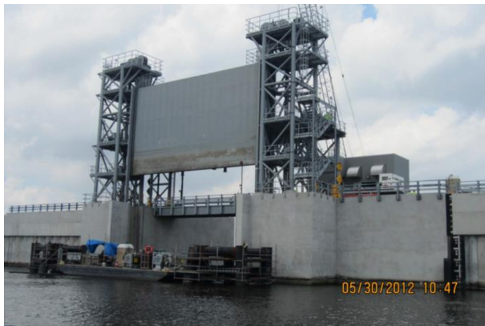
Figure 9-13. Inner Harbor Navigation Canal storm surge barrier gate leaf and tower
