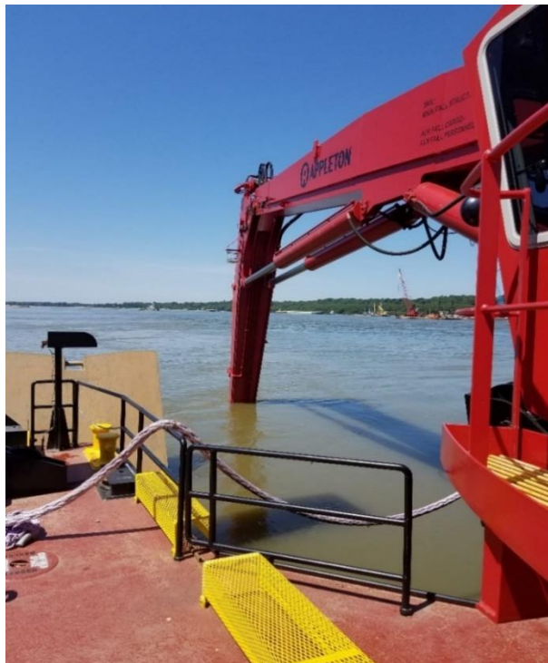
Figure 24–6. Wicket lifter crane at Olmsted raising manual wicket gate
