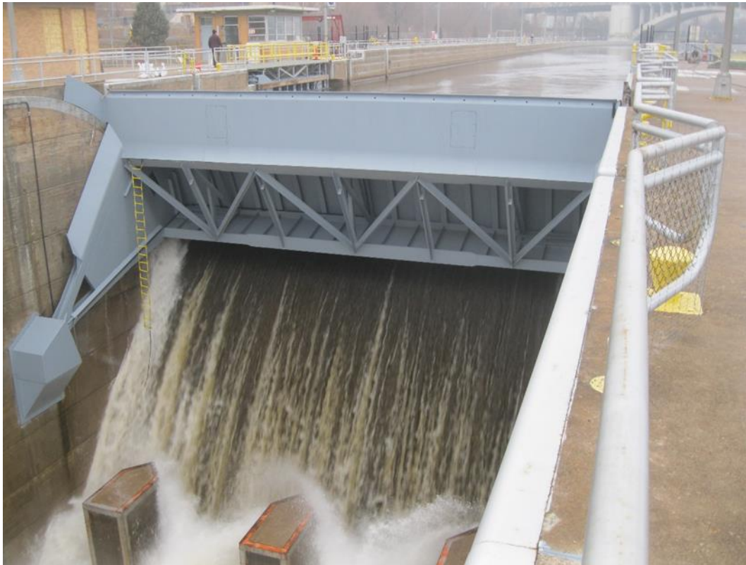
Figure 14–2. Upper St. Anthony Falls Lock tainter gate passing flood flows through lock chamber
