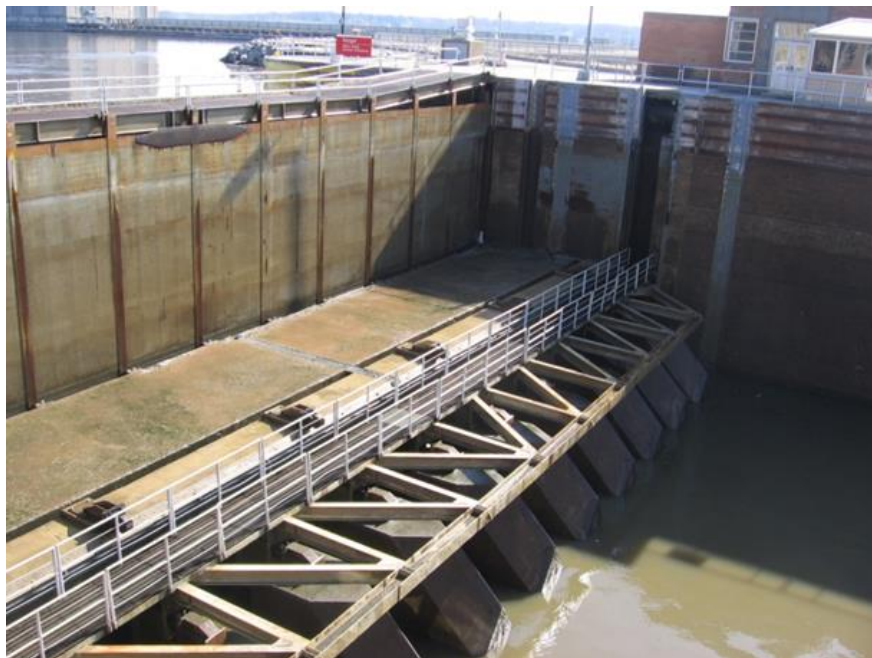
Figure 9–9. Single-leaf emergency gate
