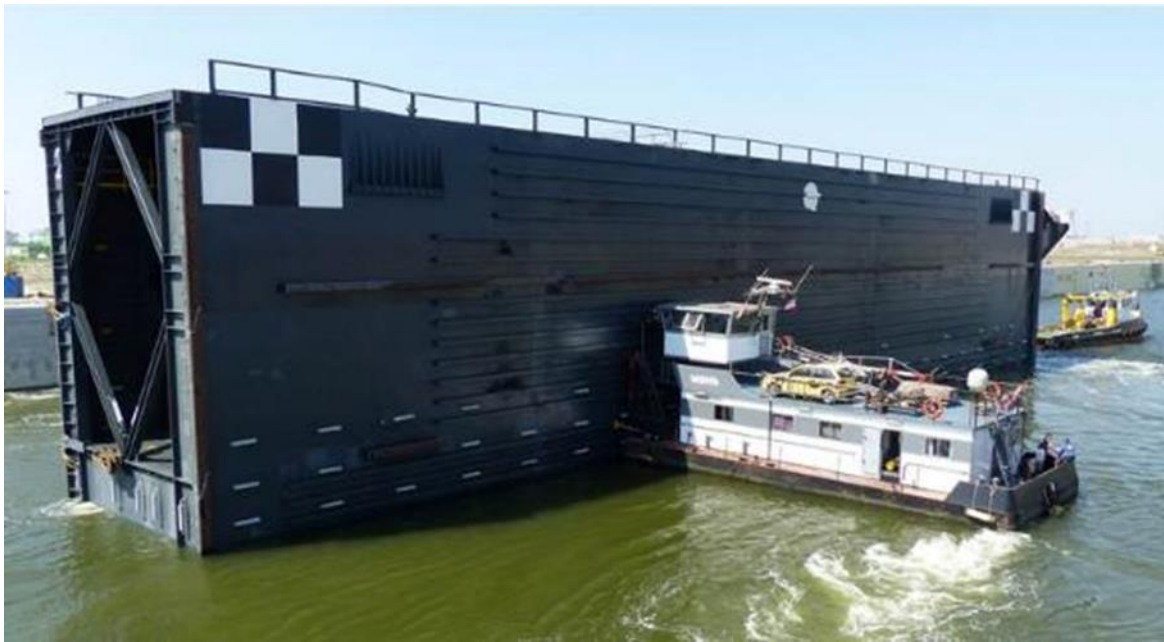
Figure 10–11. New Kieldrecht Lock rolling gate being floated into place (courtesy Vlaamse Overheid)
