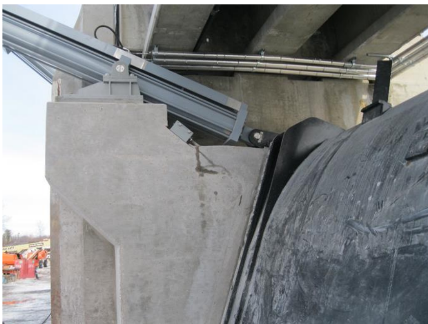
Figure 11-24. Hydraulic cylinder connection detail, Coon Rapids Dam
