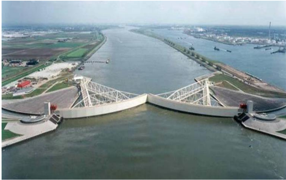
Figure 10–1. Buoyant sector gates of the Maeslant Barrier, Netherlands, in closed position (courtesy of R.A. Daniel, Rijkswaterstaat, and Hollandia)
