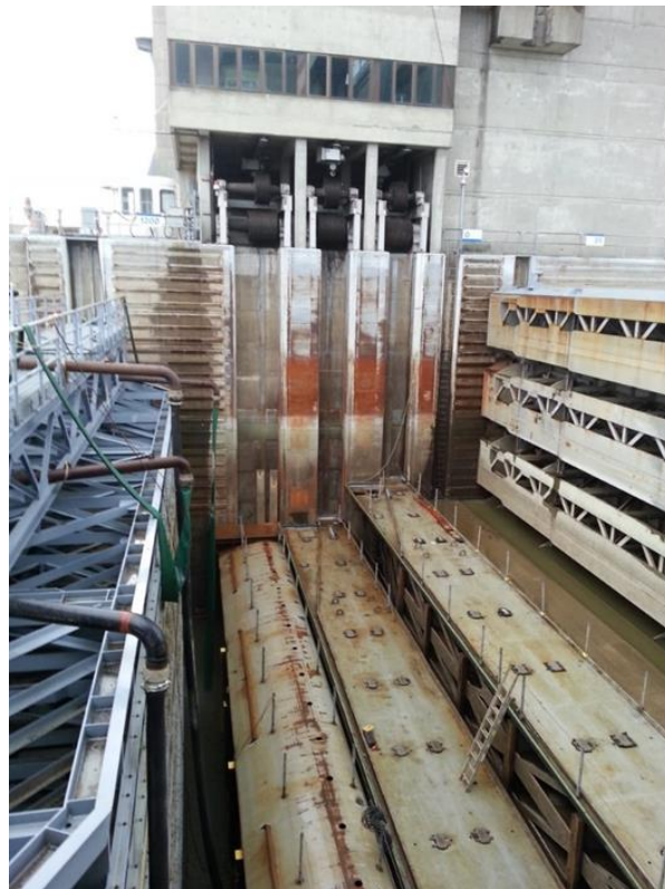
Figure 9–5. Multiple-leaf vertical lift gate, Mel Price Lock
