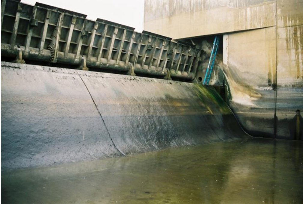
Figure 11–22. Hinged crest gate, torque tube-style (viewed from the downstream side)
