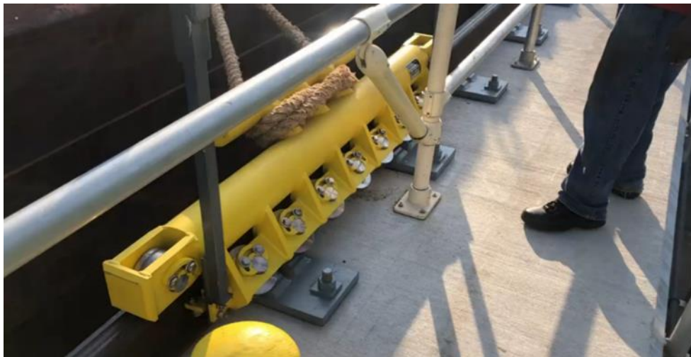
Figure 12-15. Lock and Dam 6 – towing bitt with horn assembly at 45 degree upward
