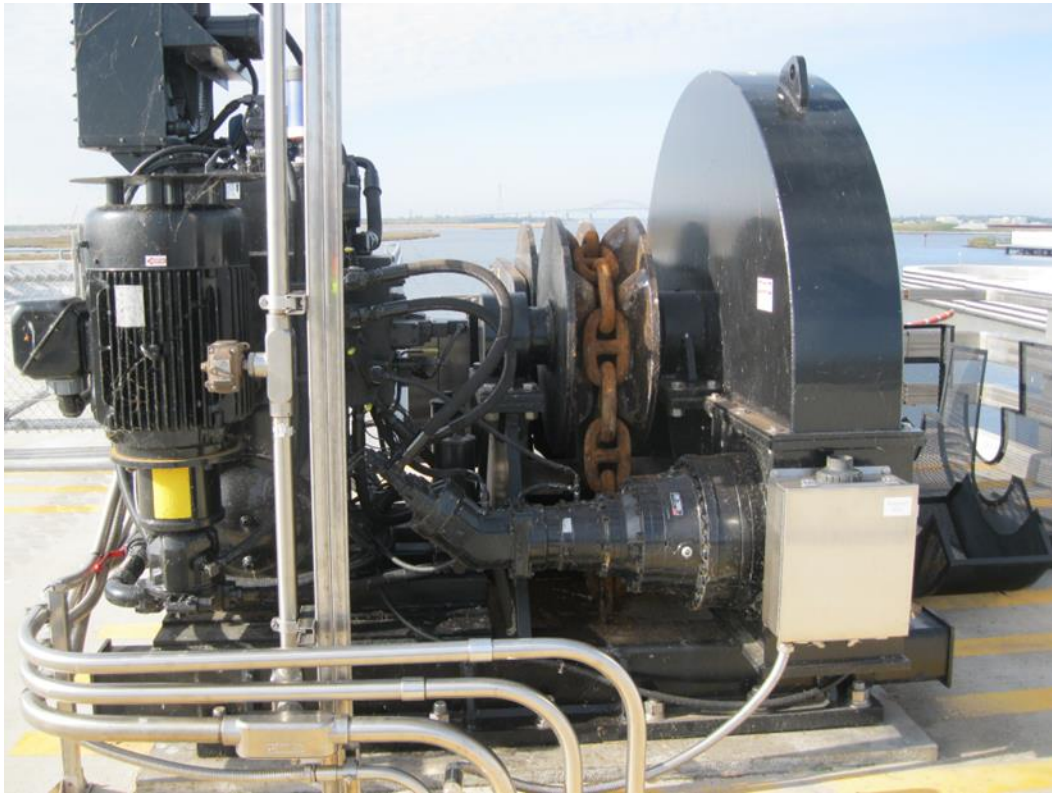
Figure 10–6. Winch system for Inner Harbor Navigation Canal barge gate
