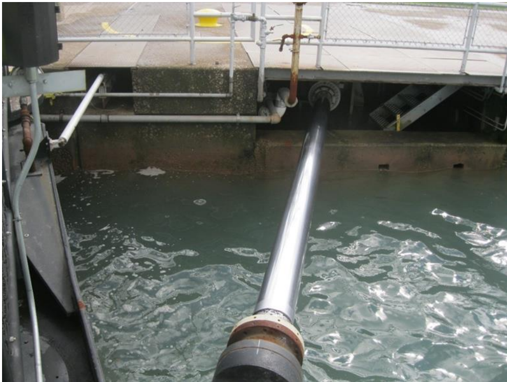
Figure 5–4. Hydraulic cylinder for Soo Locks Poe Lock miter gate
