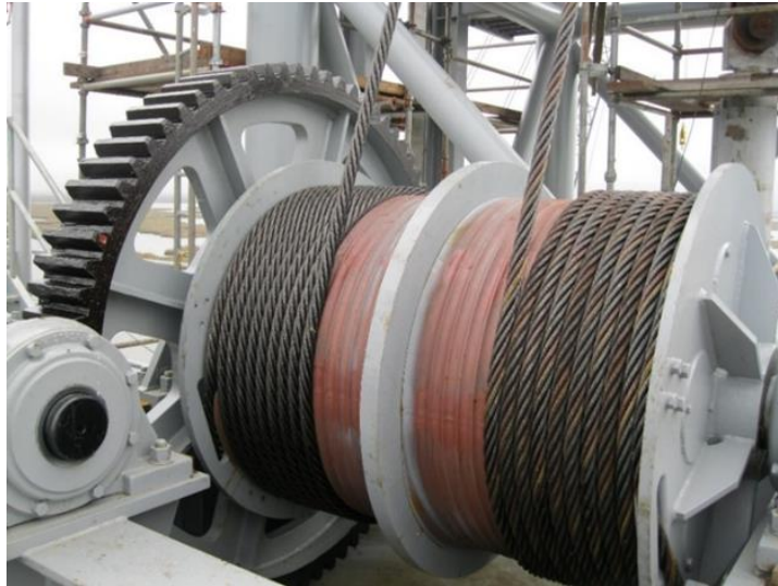
Figure 9-12. Inner Harbor Navigation Canal storm surge barrier gate machinery
