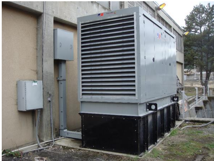
Figure 15–8. Standby diesel generator on sub-base fuel tank
