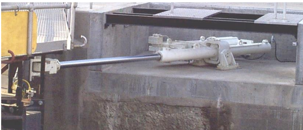
Figure 6-10. Self-contained actuator – USACE, Pittsburgh District
