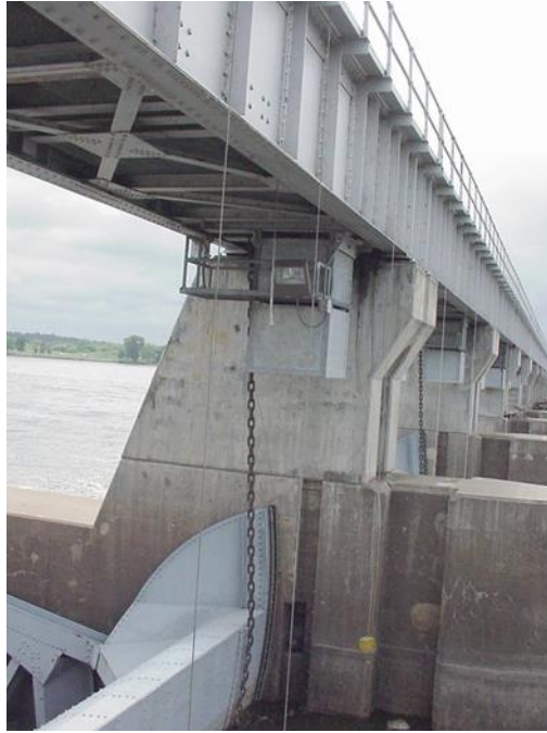
Figure 2-27. Pocket wheel hoisting assembly
