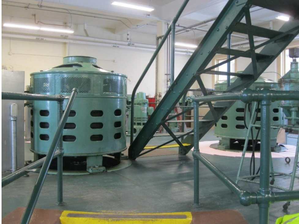
Figure 22–5. Davis Well pump motors on operating deck
