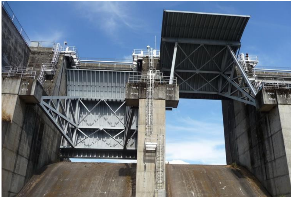
Figure 11–1. Conventional spillway tainter gate
