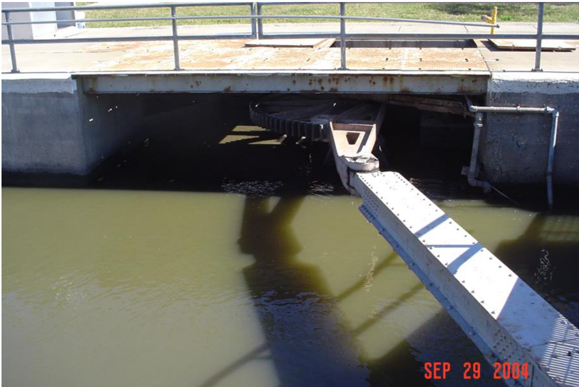
Figure 6–4. LaGrange Lock, Illinois River, Ohio linkage
