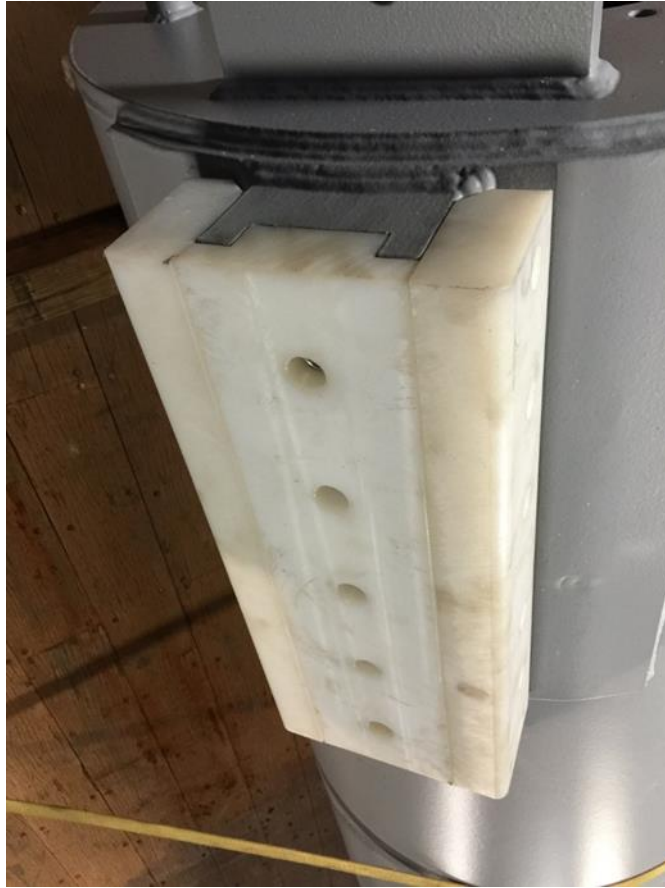
Figure 12–38. Cheatham Lock – ultra-high molecular weight polyethylene guides for floating mooring bitts
