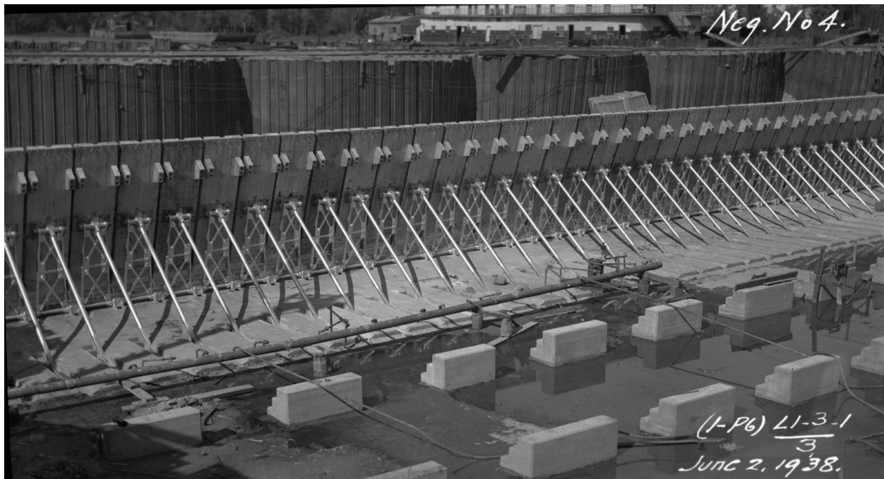
Figure 24–9. Lagrange wicket gates
