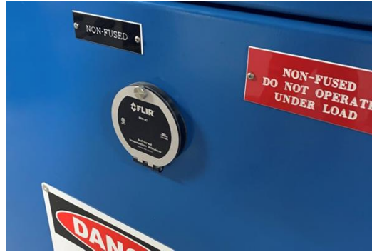
Figure 15–17. Inspection window in 15-kV disconnect switch
