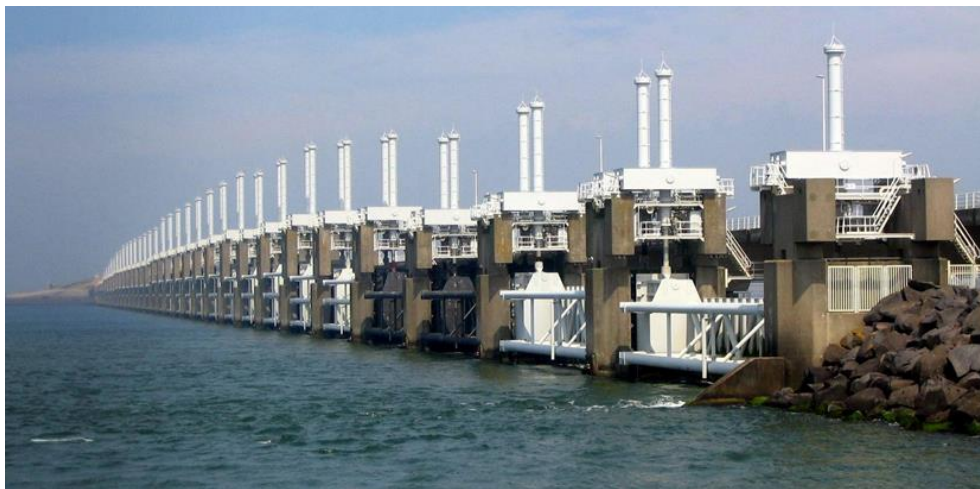
Figure 9–14. Direct-connected hydraulic vertical storm gates, Eastern Scheldt Storm Surge Barrier, the Netherlands (R.A. Daniel and Rijkswaterstaat)
