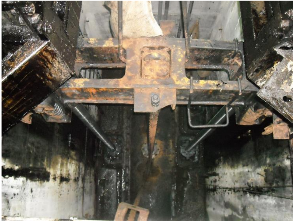
Figure 8–11. Chittenden Lock Stoney valve drive
