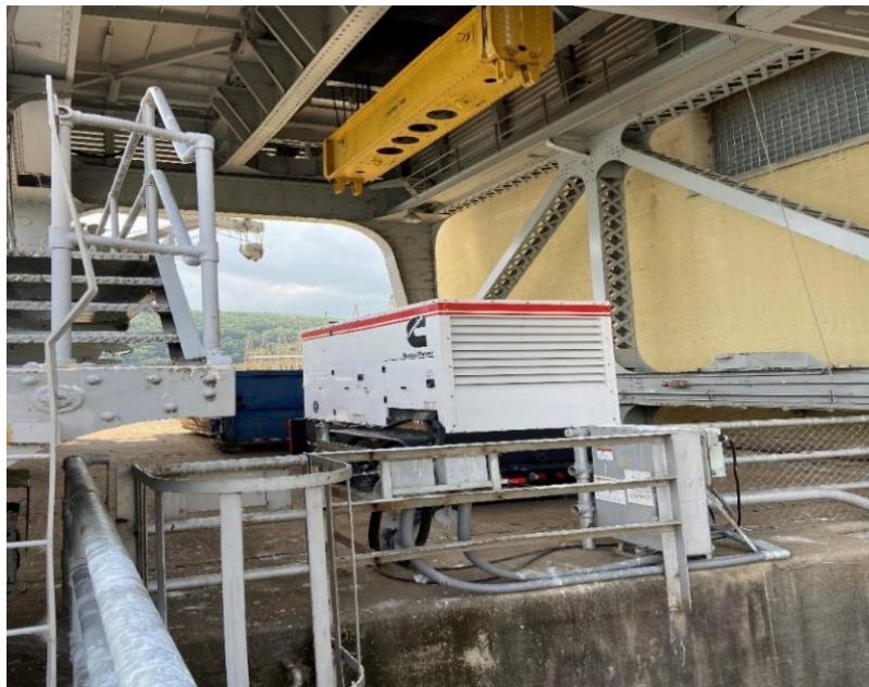
Figure 26–2. Guntersville backup generator for powerplant intake/dam spillway crane
