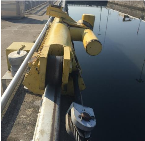
Figure 12–25. Old Hickory Lock – towing bitt with adjusting rod for tensioning wire rope
