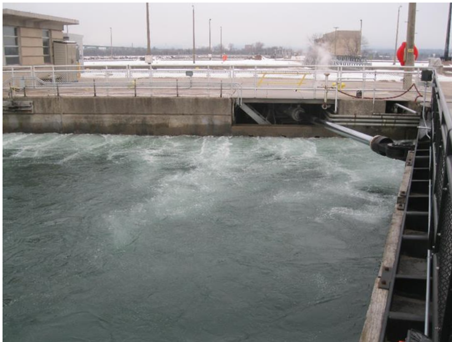
Figure 14–4. Poe Lock air bubbler system in operation
