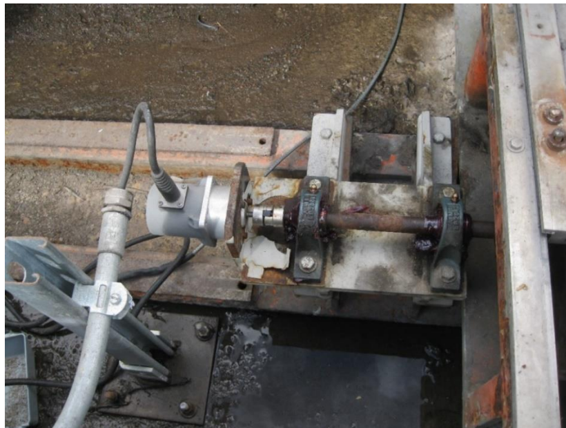
Figure 5–7. Soo Locks miter gate encoder
