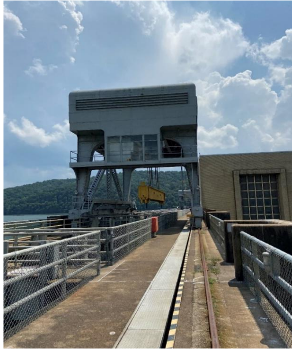
Figure 26-3. Gunter'sville Project, trench for electrical conduits of the powerplant intake/dam spillway crane
