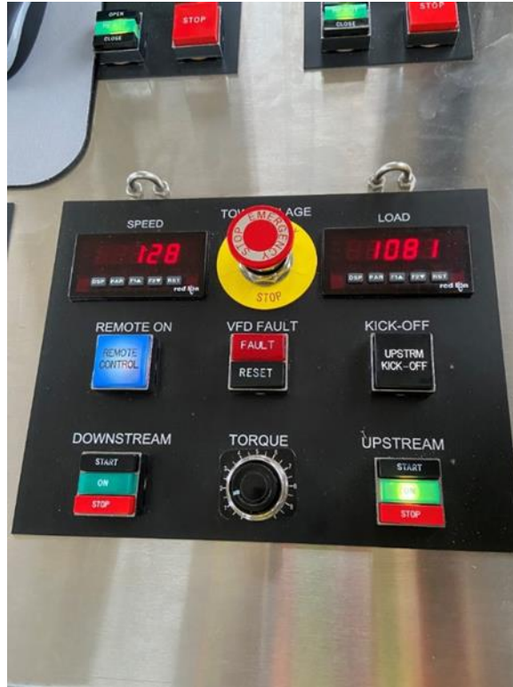
Figure 12–28. Barkley Lock – tow haulage control at lock control shelter
