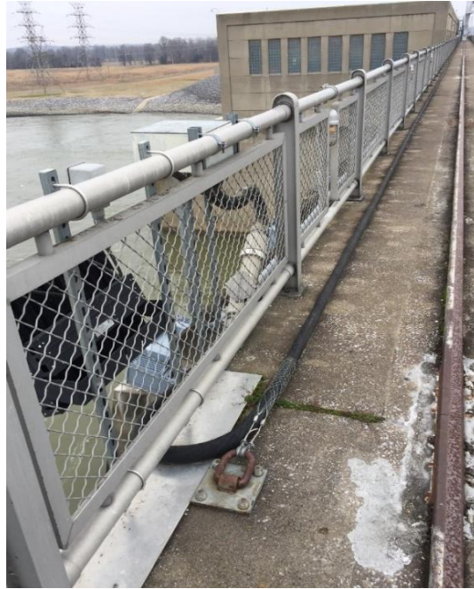
Figure 26–5. Barkley Project, anchored point for electrical conduit of the power reel for the powerplant intake/dam spillway crane
