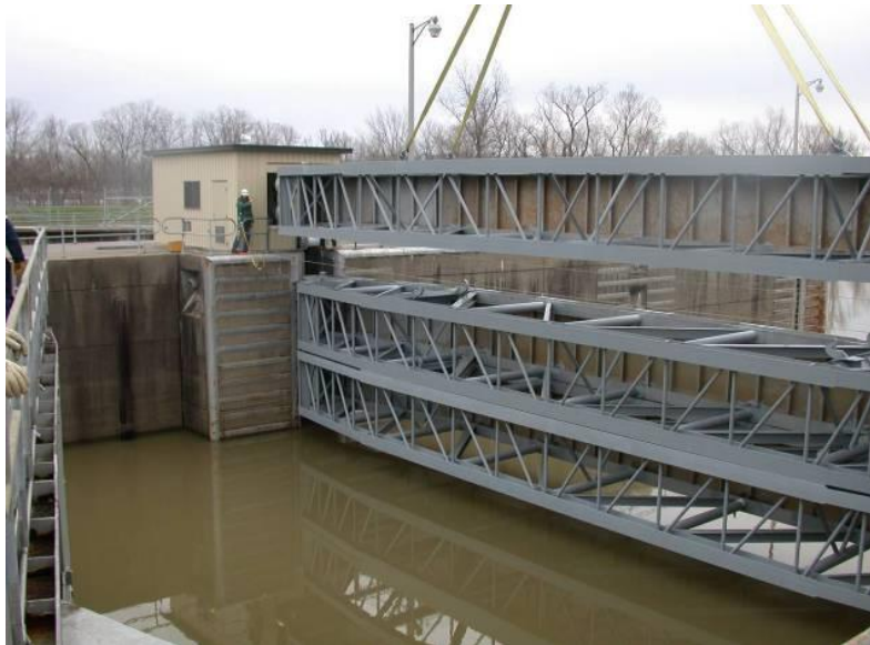
Figure 26–11. Emergency bulkhead system, Old River Lock between Mississippi and Atchafalaya rivers
