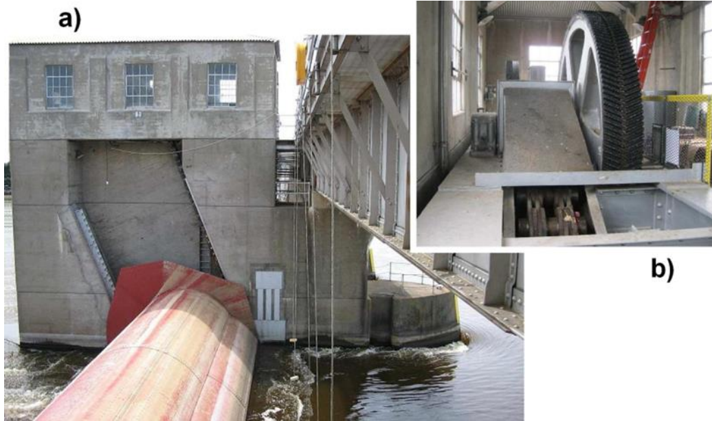
Figure 11–28. Roller gates on the Mississippi, drive machinery: a) driven end and machine room on pier; b) view inside machine room
