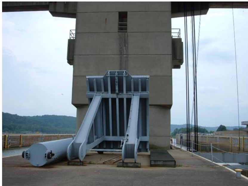
Figure 8–3. Reverse tainter valve
