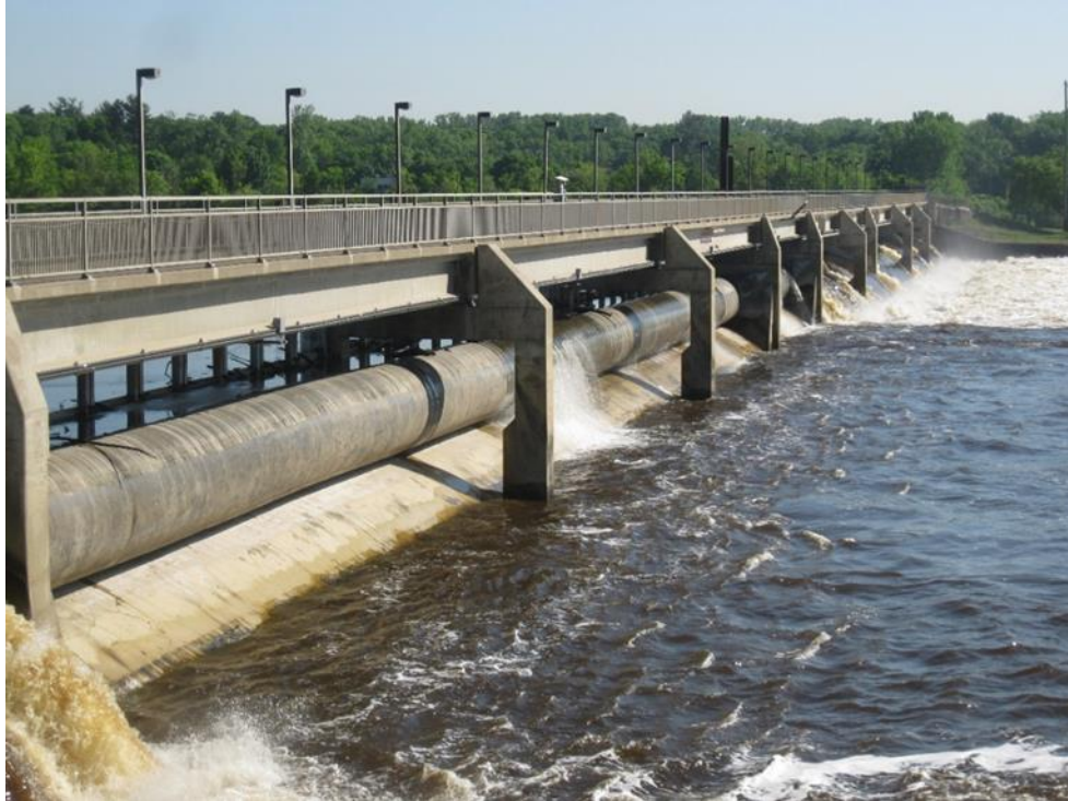
Figure 13–5. Old Coon Rapids Dam rubber gates on Mississippi River
